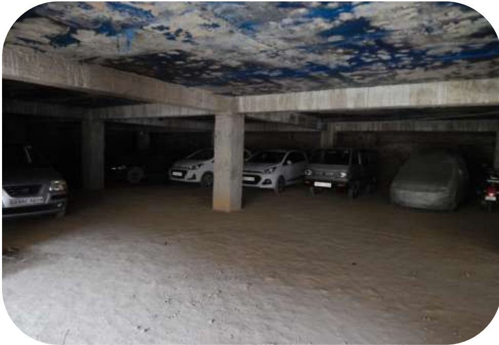
View of parkinglot inside the building
