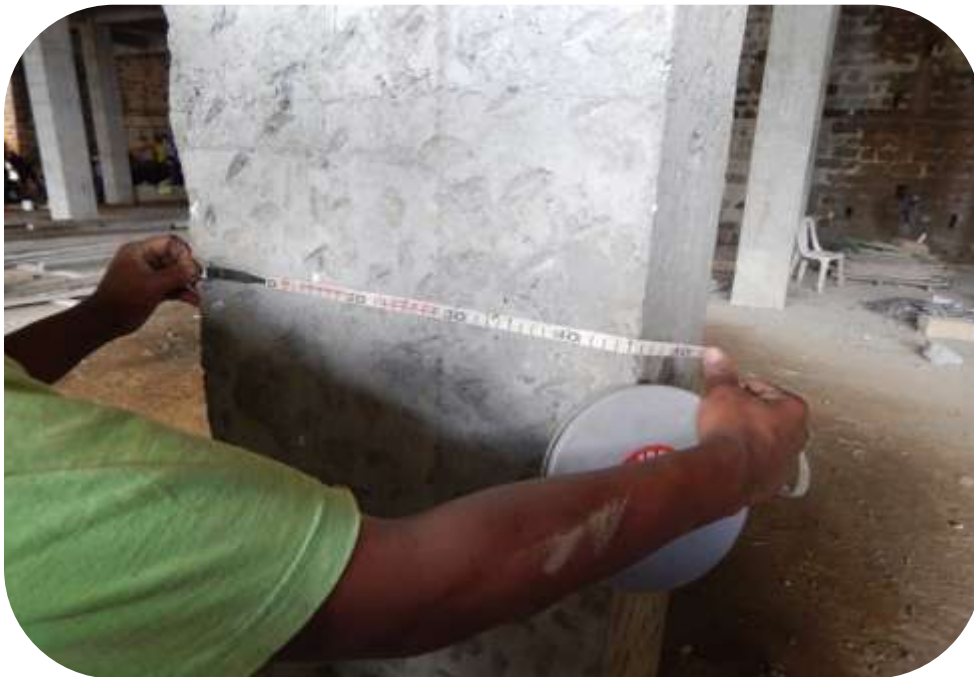
Consultant measuring the size of column
