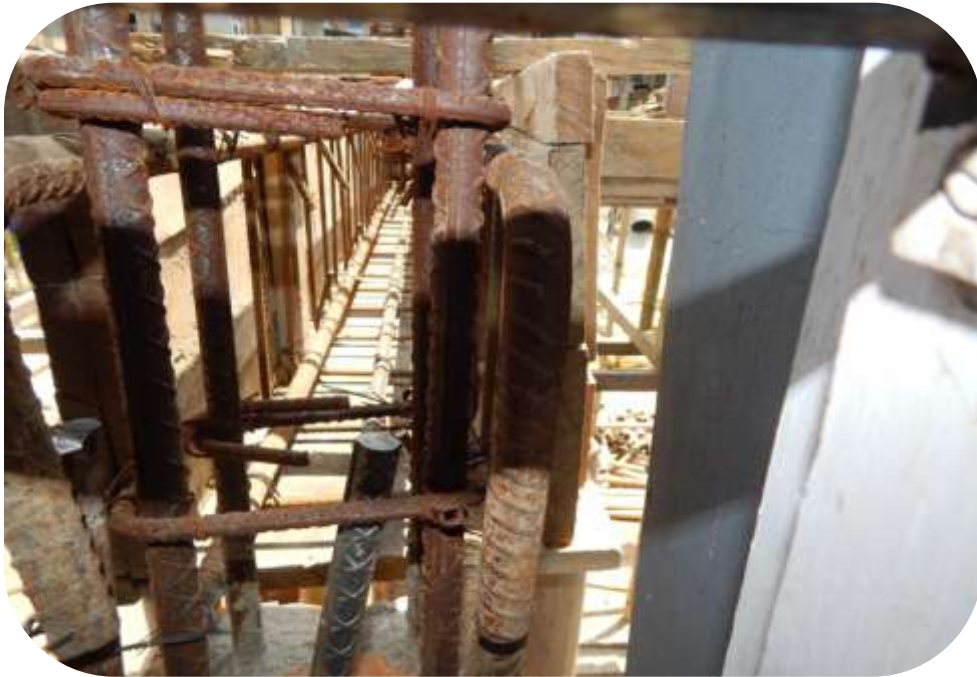
Lapping of reinforcement
