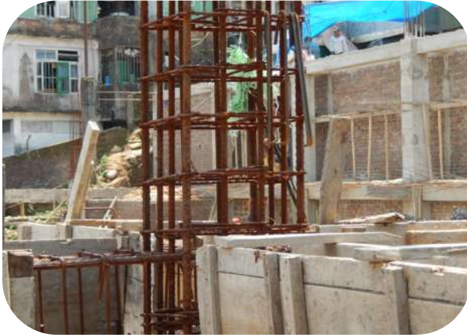
View of reinforcement used at site
