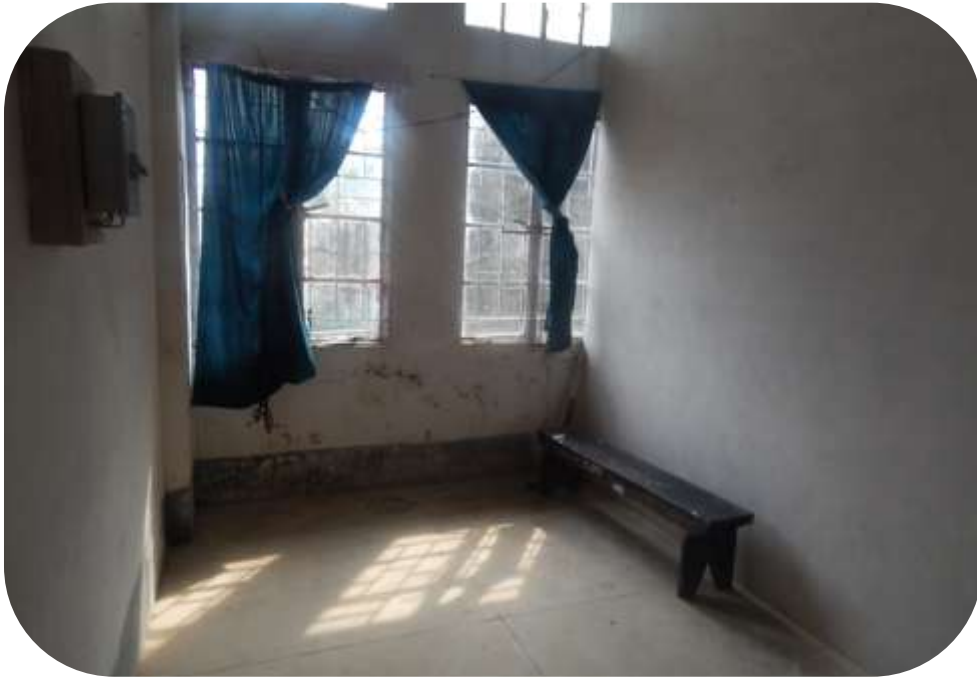
View of control room
