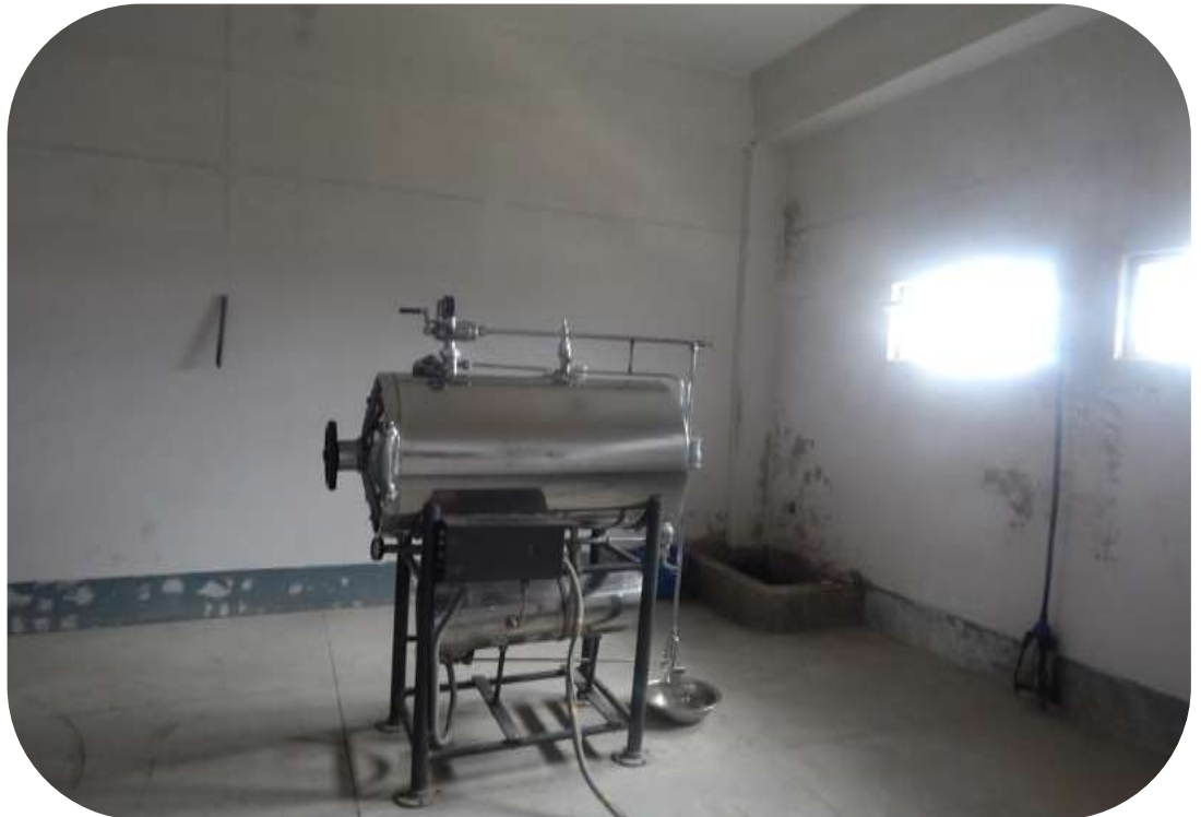
View of room to be used for CT Scan
