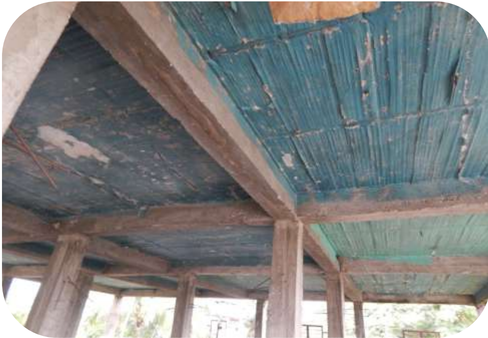
View of columns, beams and Slab
