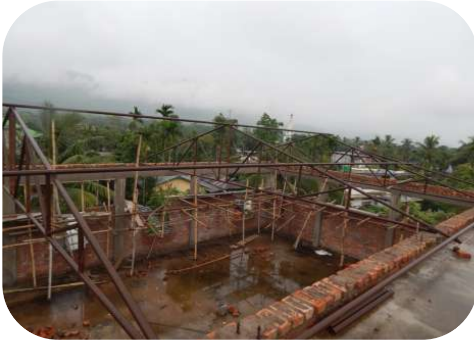
View Truss work
