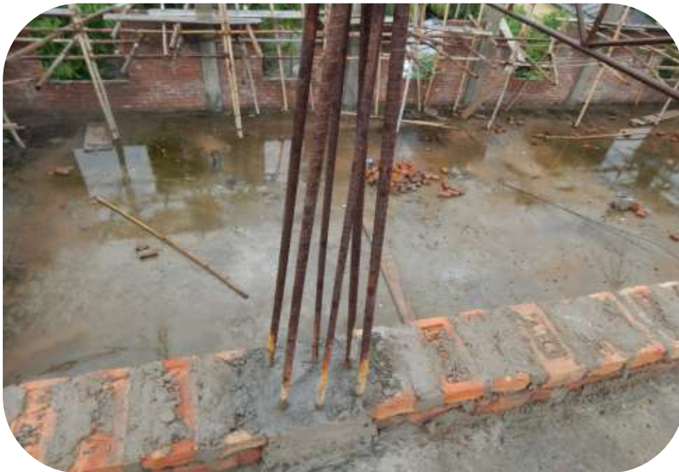
View of reinforcement
