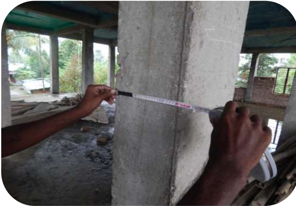
View of column
