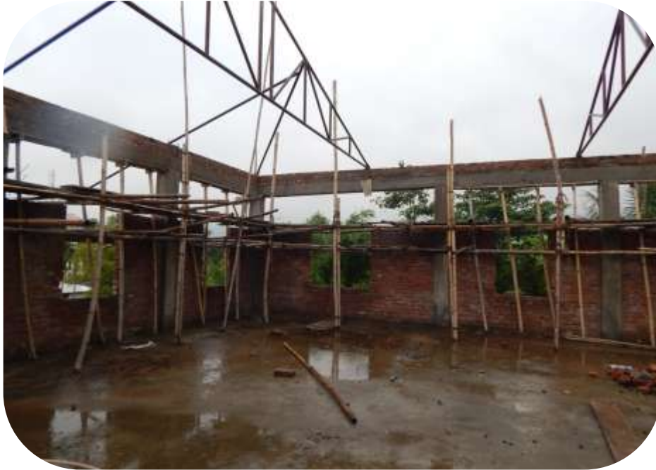
View of truss works
