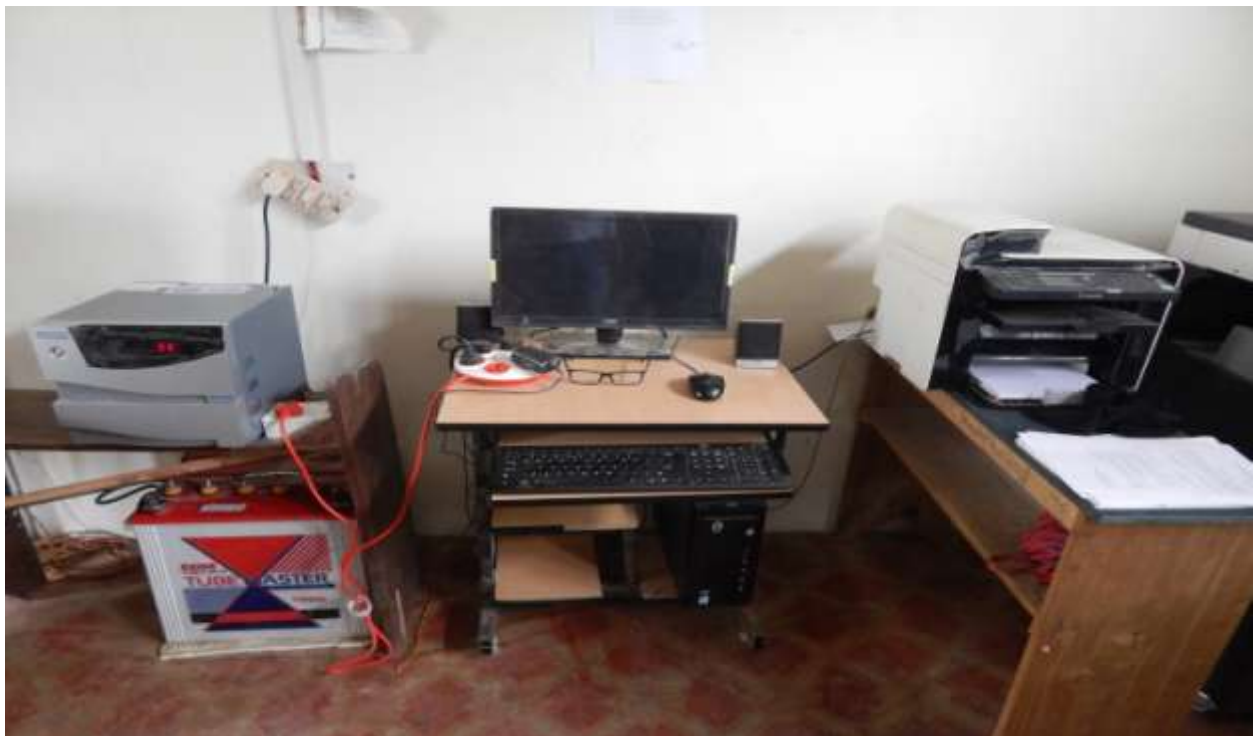
View of UPS,Desktop PC at Government Mamit High School at Mamit,Mizoram
