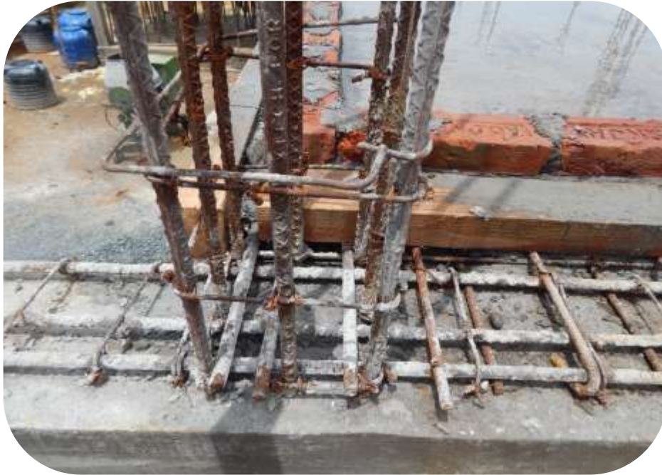
View of reinforcement used in Meluri
