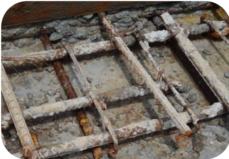
View of beam and Slab in Meluri
