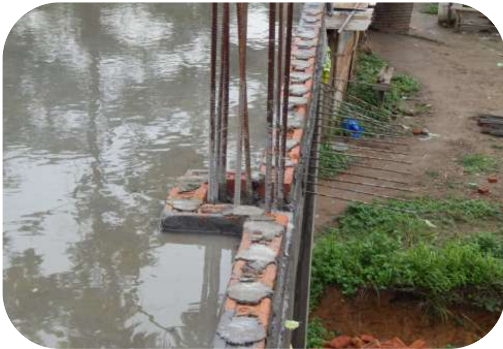
View of reinforcement in Medziphema
