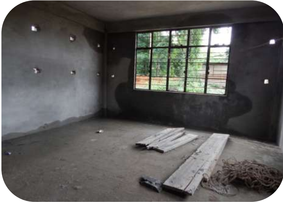
Inside the building
