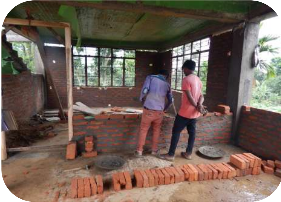
View of Brick work
