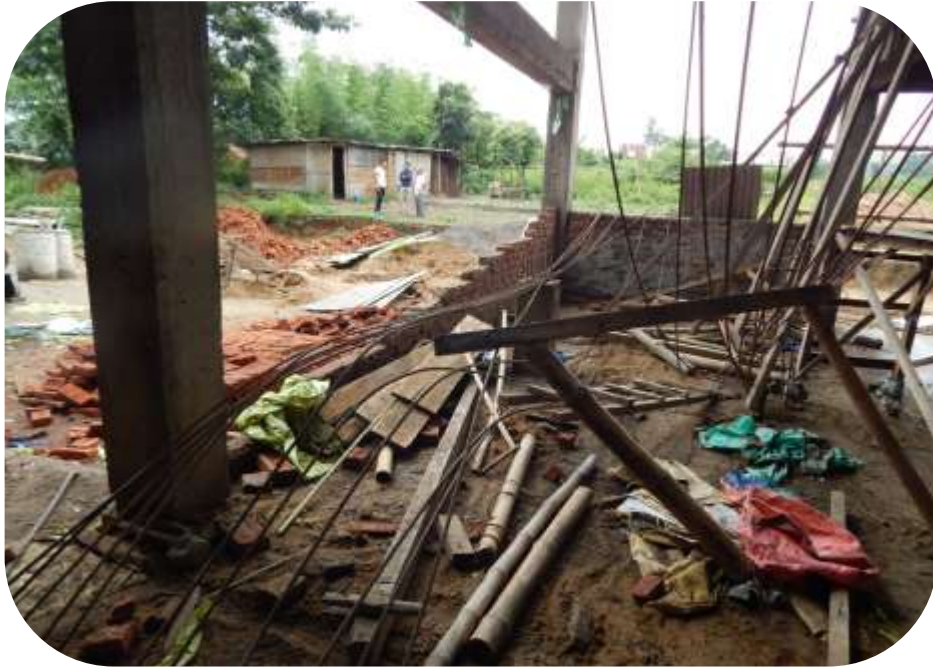
work on ramp
