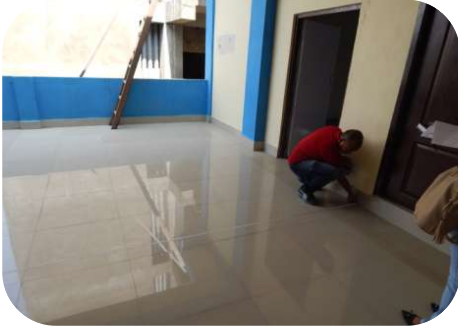
Consultants measuring the area of the Building
