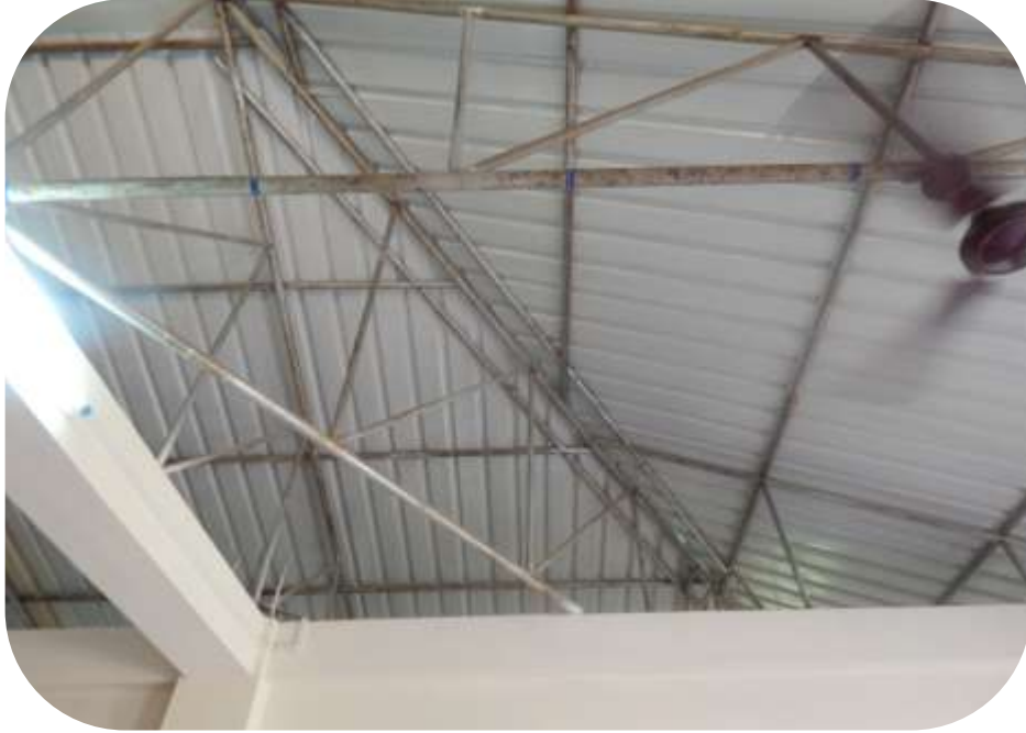
View of Truss work.
