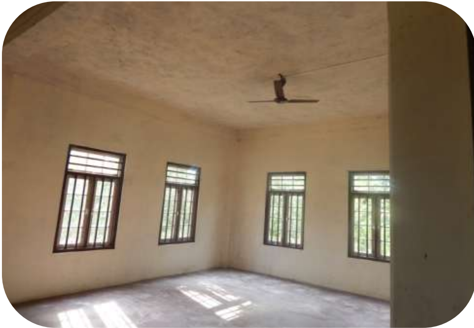
View of ceiling
