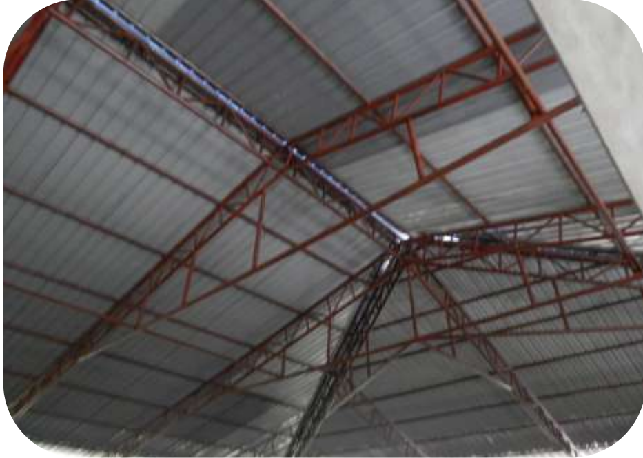
View of truss in 10m range
