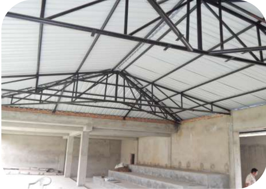
View Truss work in 50m range
