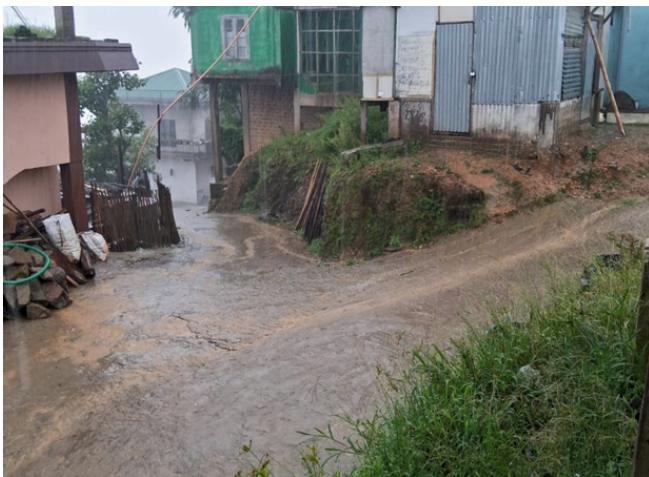
Fig. 3- Rainwater spreading all over the surface due to absence of drainage system. Muthi, May. 2024.
