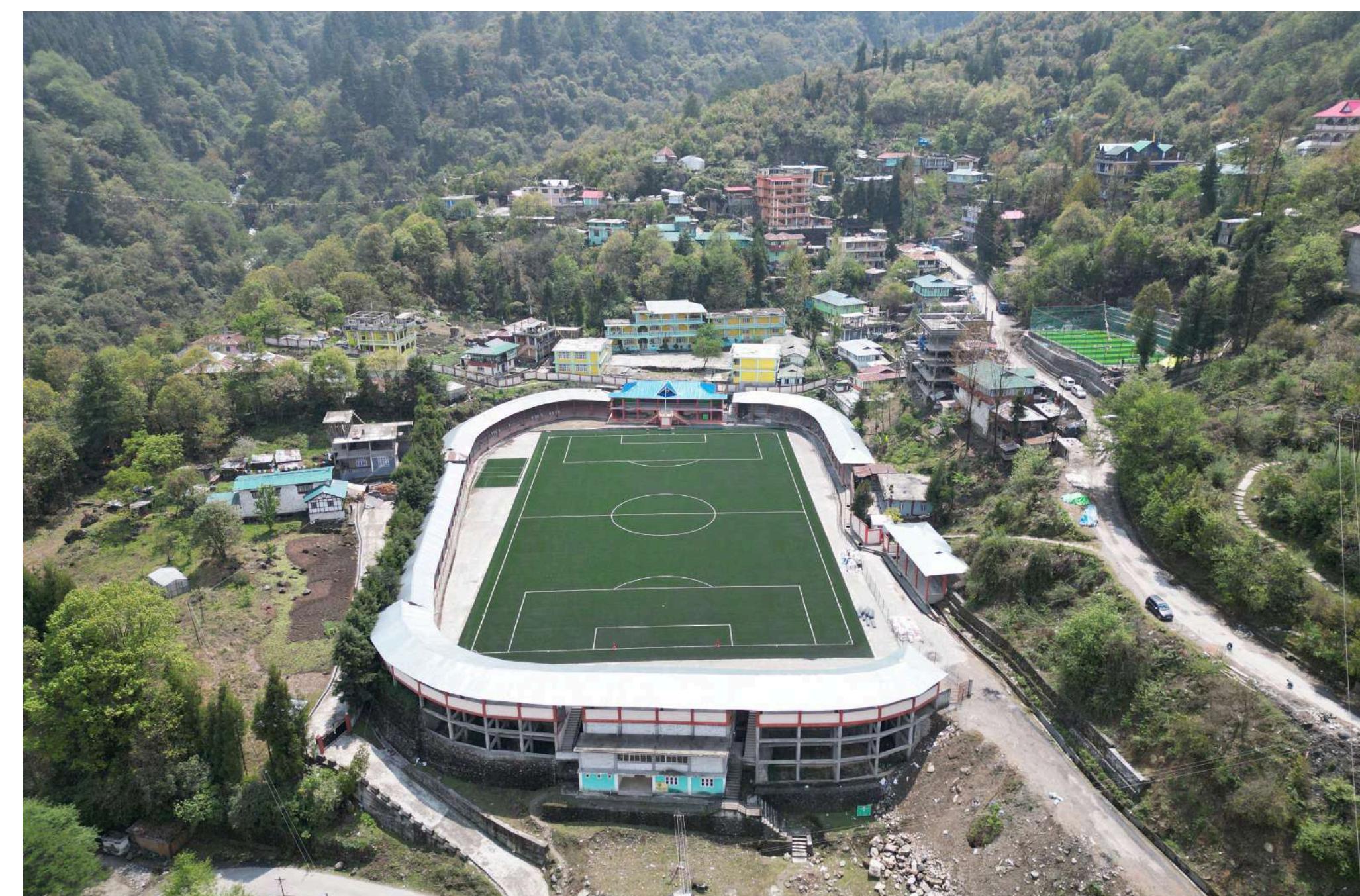
Outdoor Stadium at Jang in Tawang District
