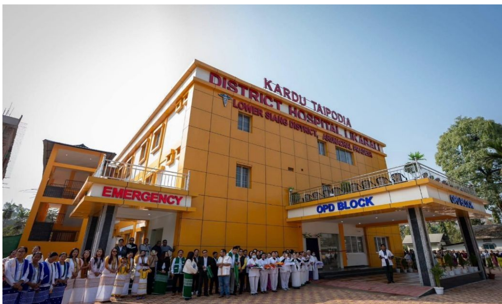
Pic: Recently completed Upgradation of District Hospital, Likabali.
