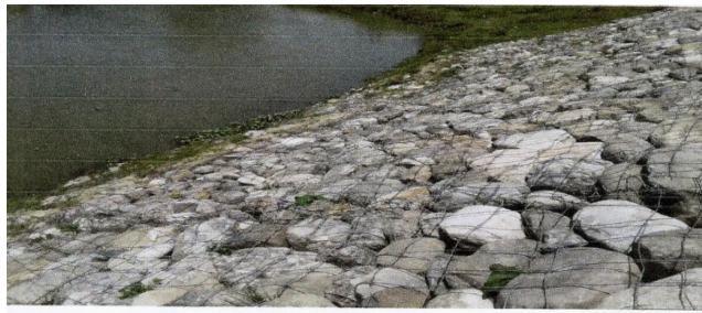
Location :- At Rajabil Village (Ch.465.00m to Ch.600.00m)
