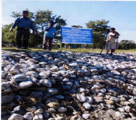
Sign Board Erected
