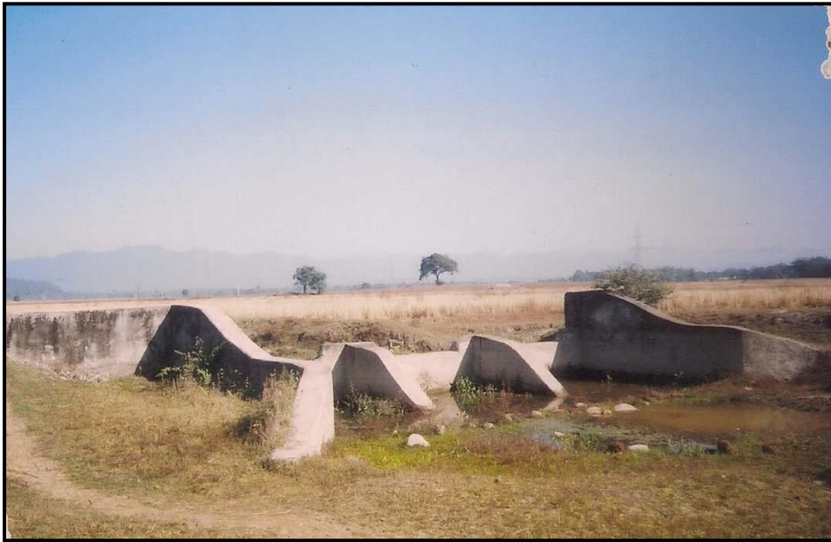
Water Harvesting Structure across Kekurajuli stream
