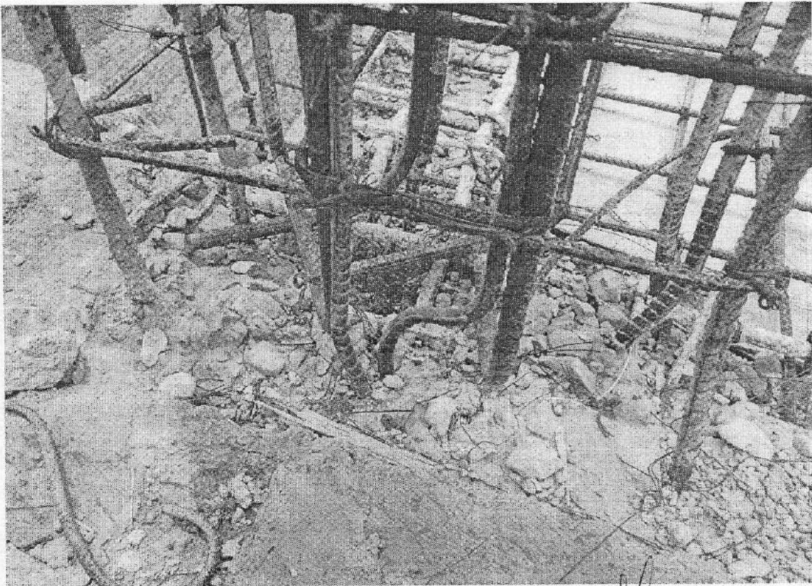
Photo of the reinforcement in columns are being bend.
