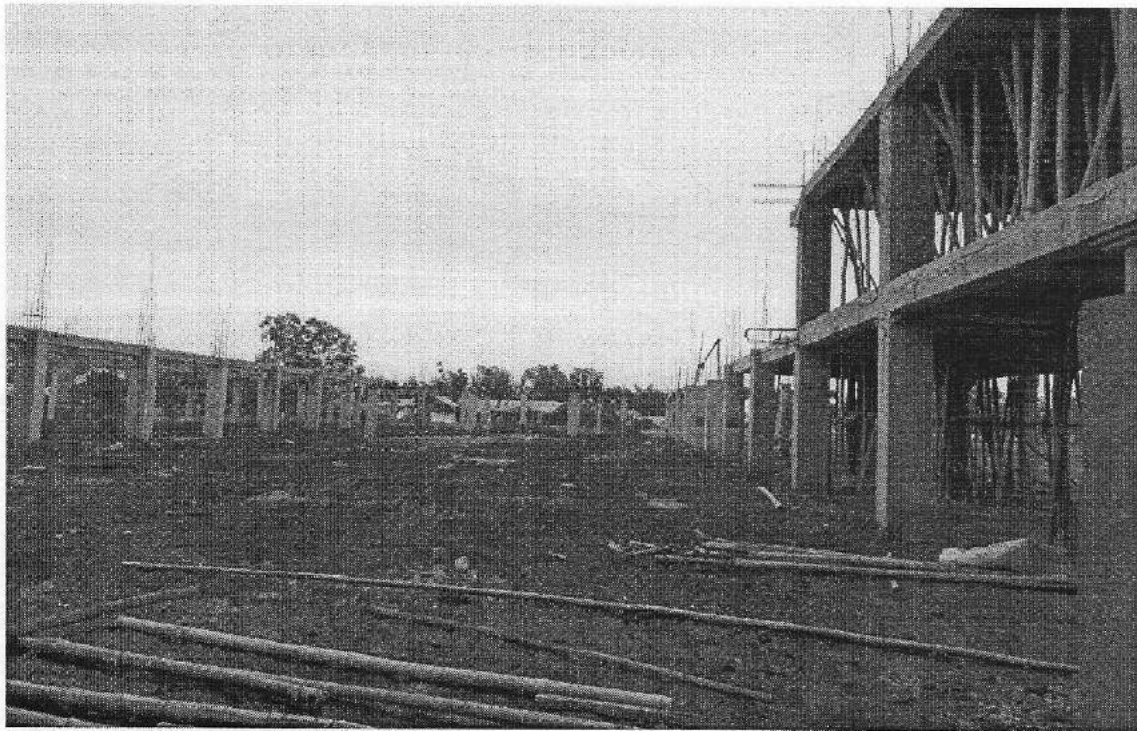
The View of the site Construction of Sainik School
