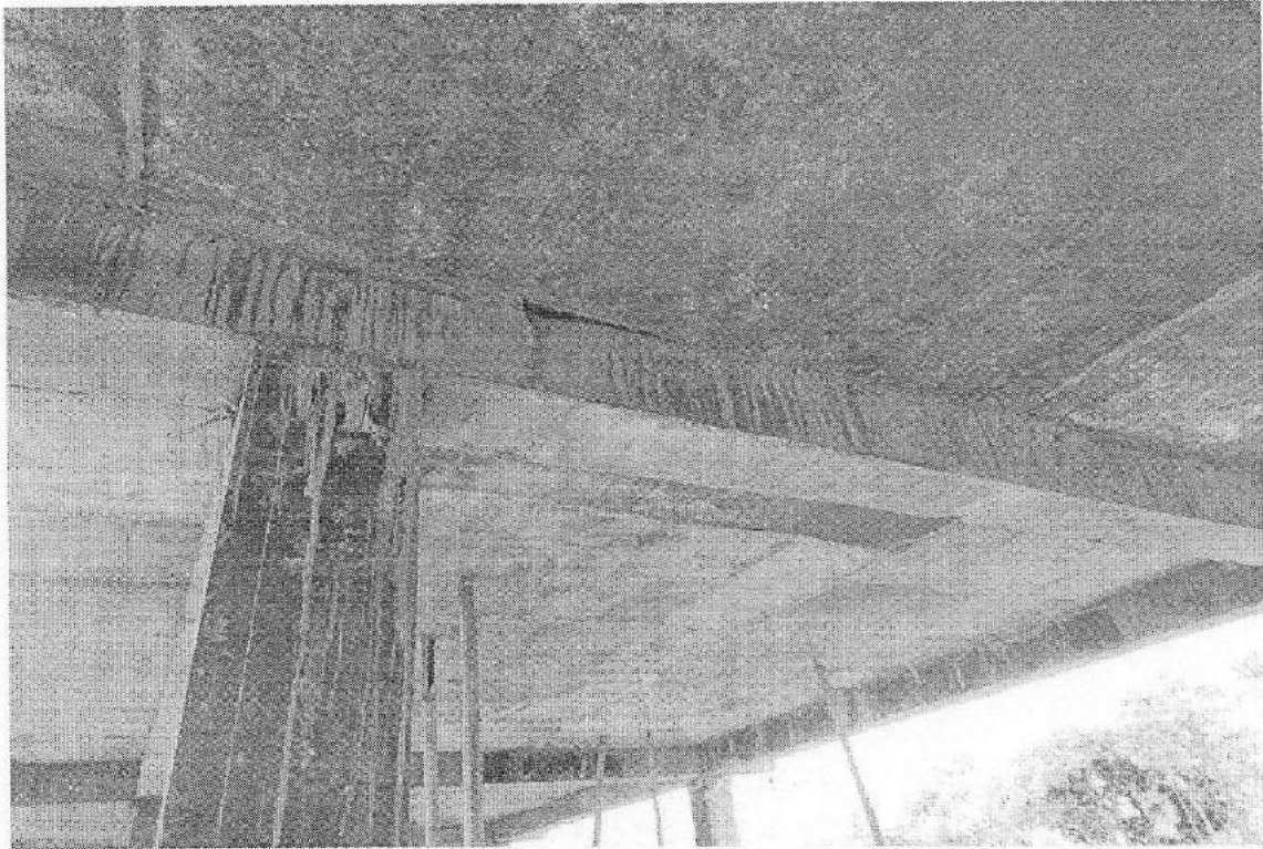
Photo of Beam
