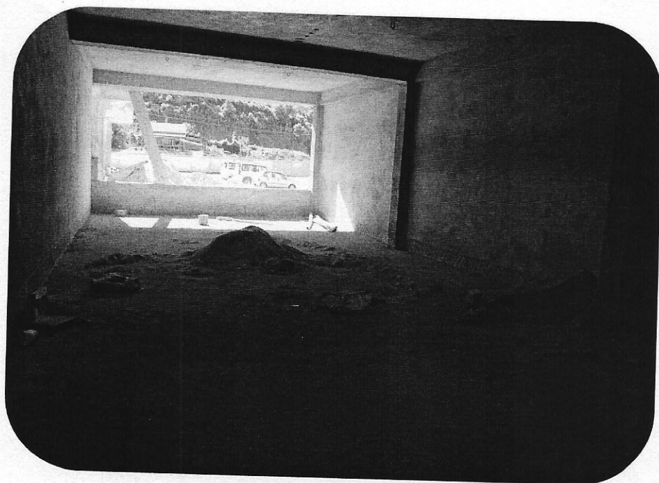
View of inside Block-A
