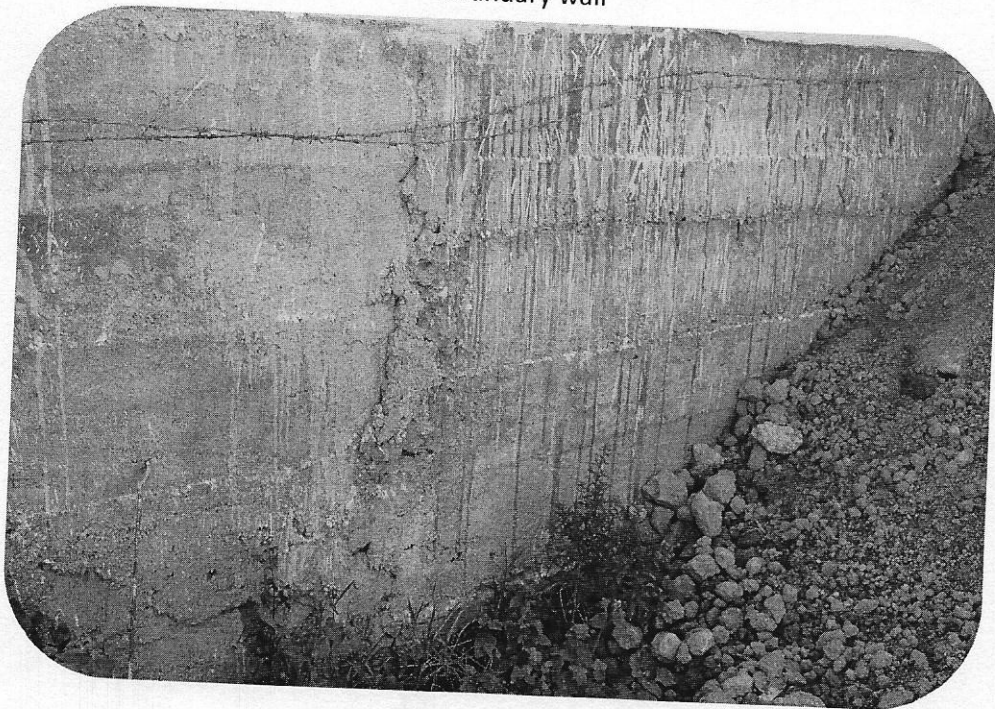
View of Retaning Wall
