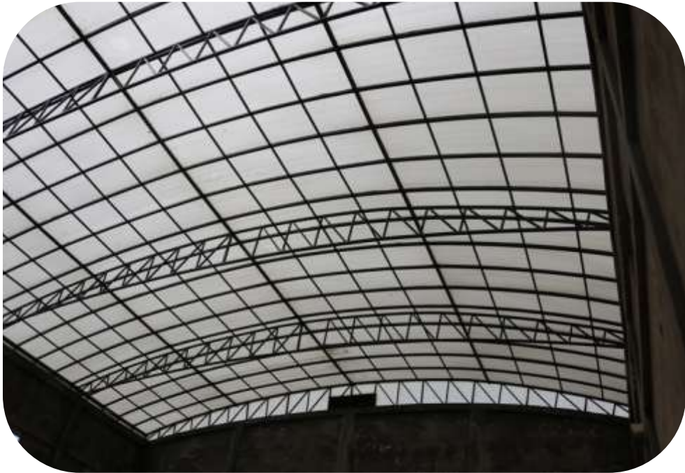
View of Truss
