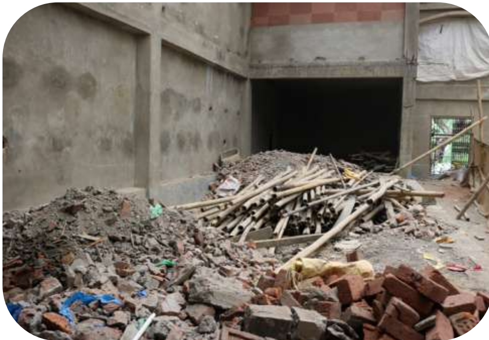
View of Stage under construction
