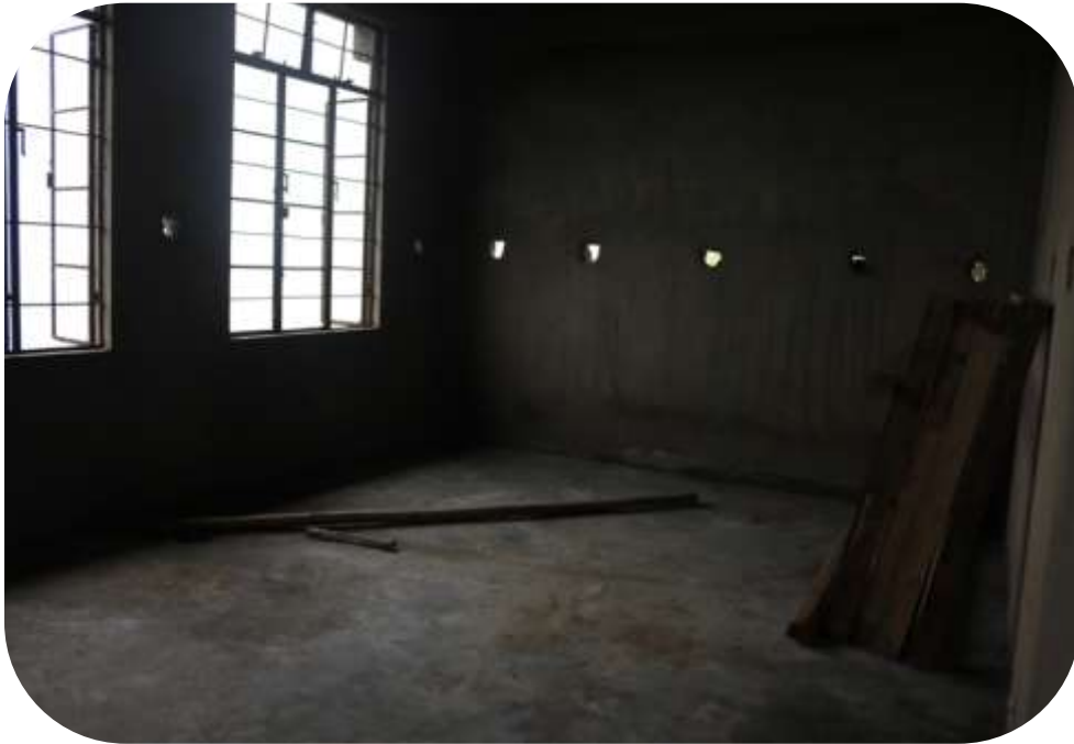
View of room inside the building
