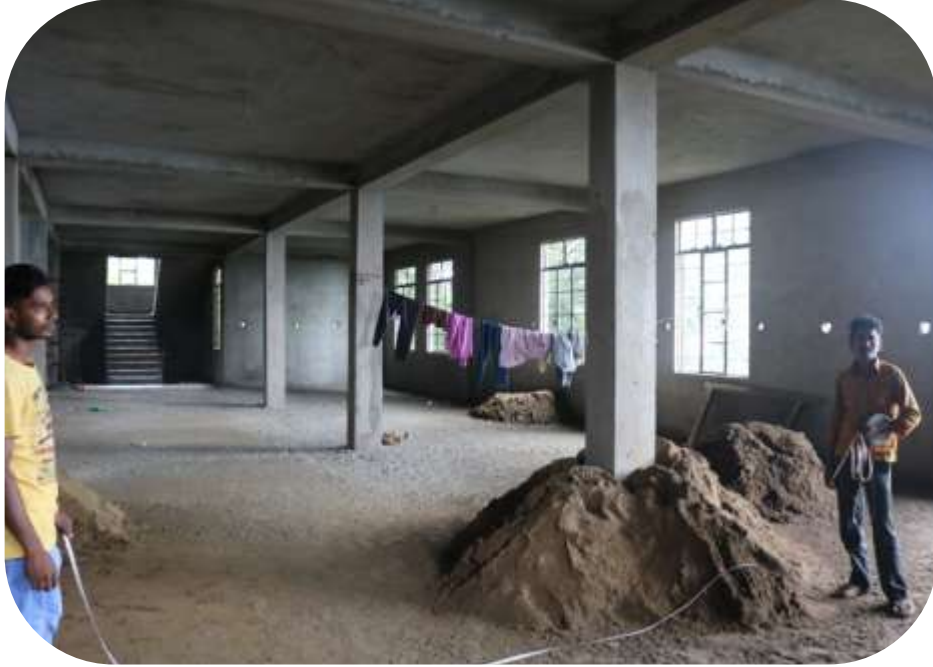
View of Library. Partition wall not yet done.
