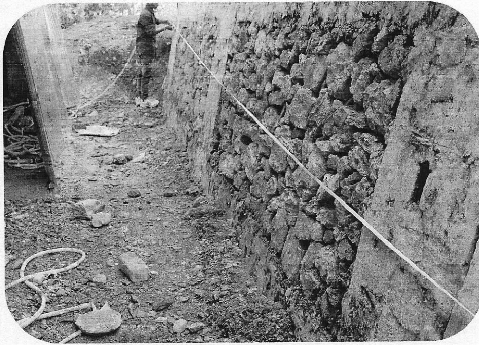
Consultant measuring the length of the wall
