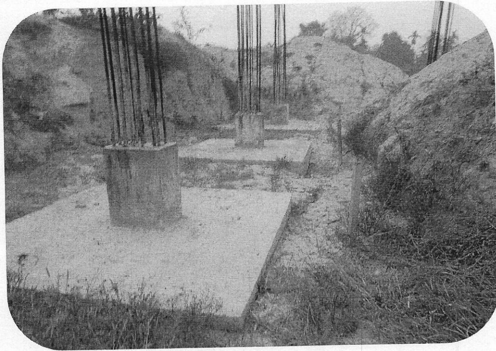
View of columns and base of footing laid over pile foundation
