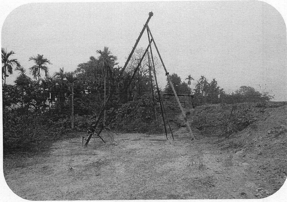
view of machine used for pile foundation.
