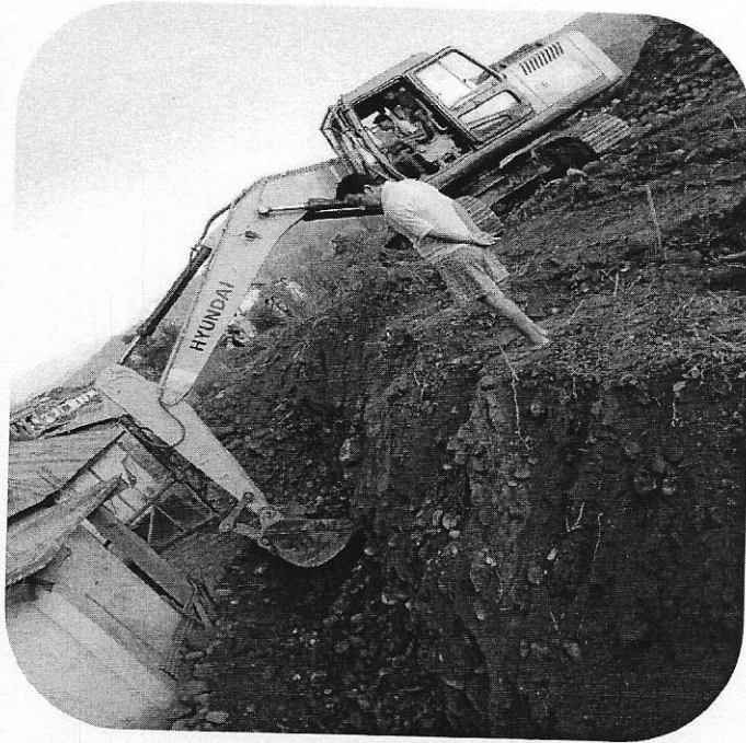
View of excavation done for retaining wall
