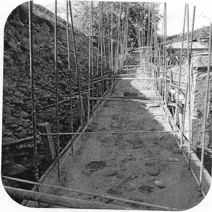
Laying of concrete for retaining wall
