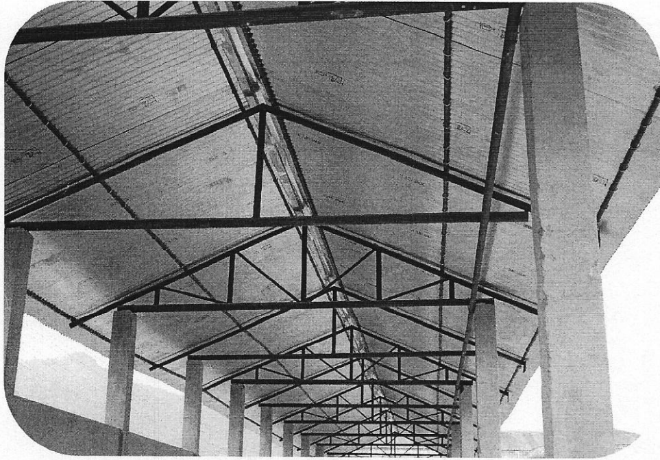
View of truss and GI sheet
