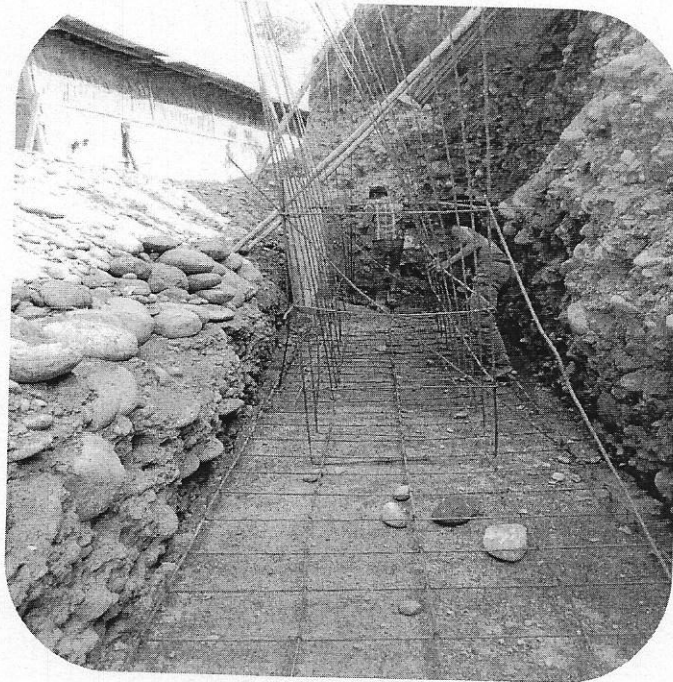
Laying of reinforcement for RCC retaining wall
