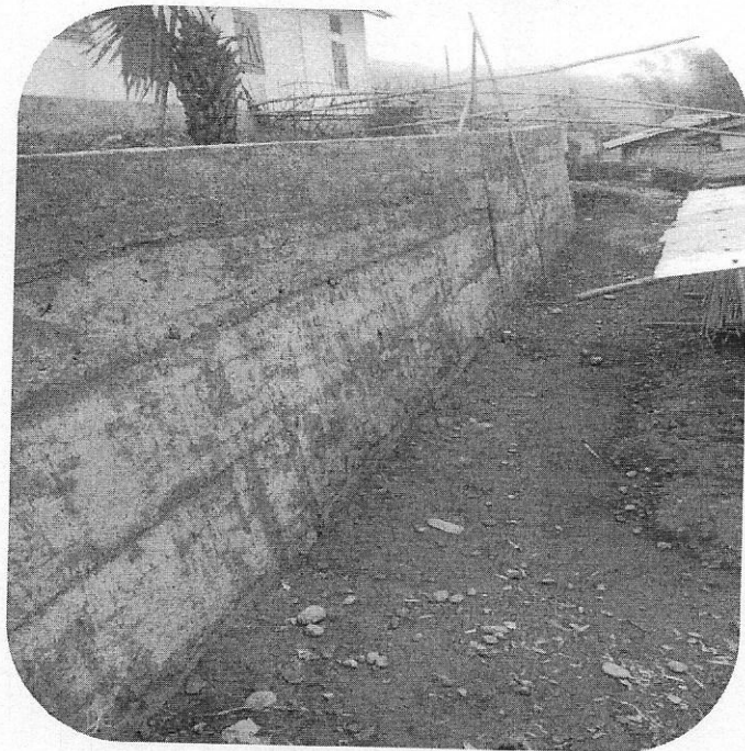
view of completed wall
