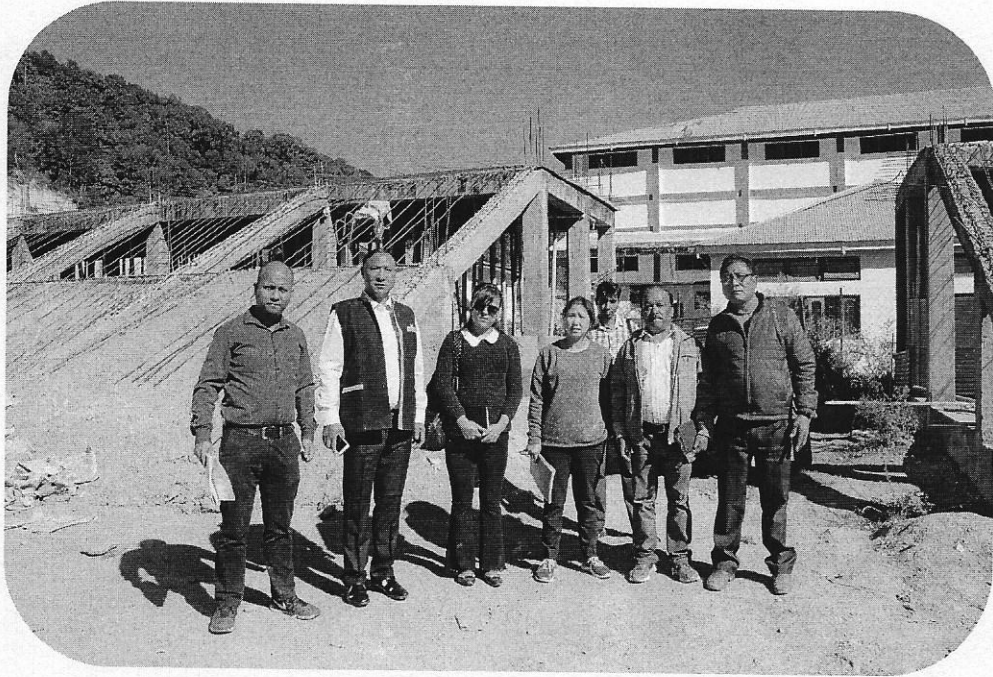
Inspection team with Implementing Agency at project site
