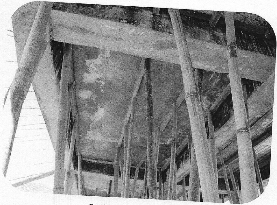
Casting of slab in progress
