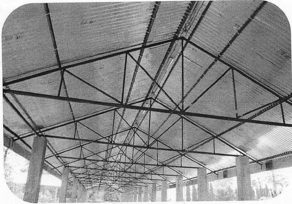
View of truss and GI sheet
