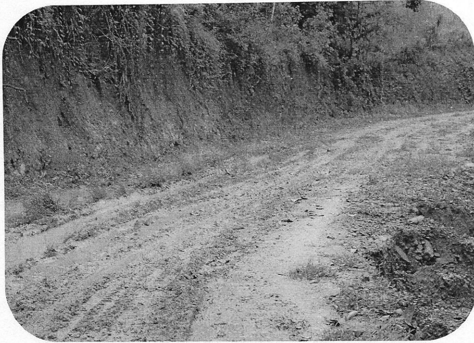
View of excavated area
