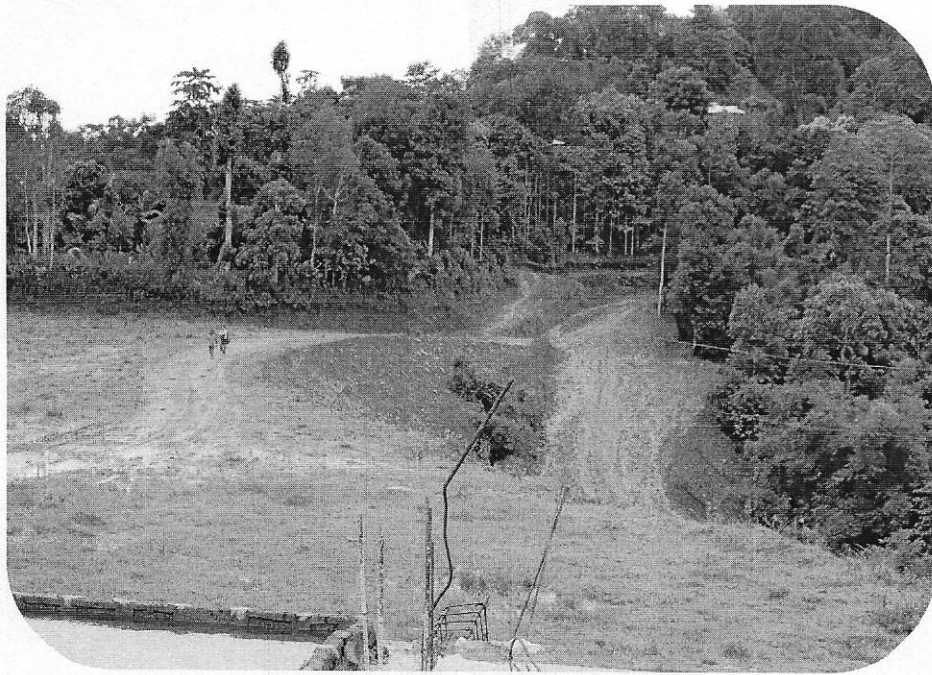
View of New road leading to the Ground
