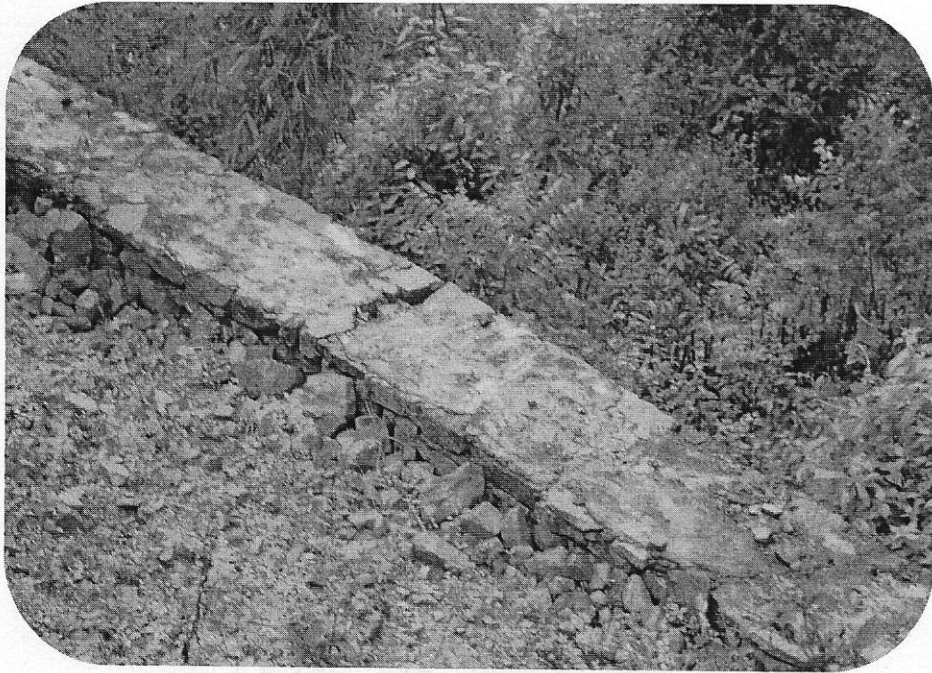
View of Retaining Wall.
