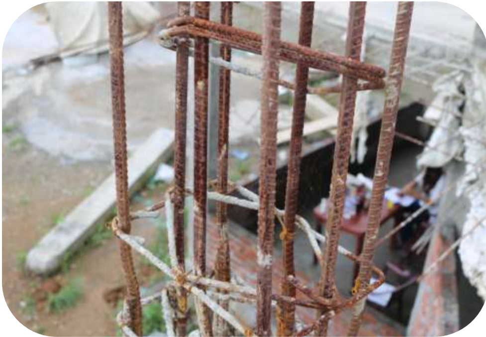
View of reinforcement used in some columns.
