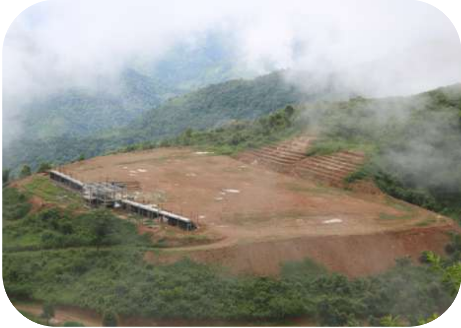
view of project site afer excavation work
