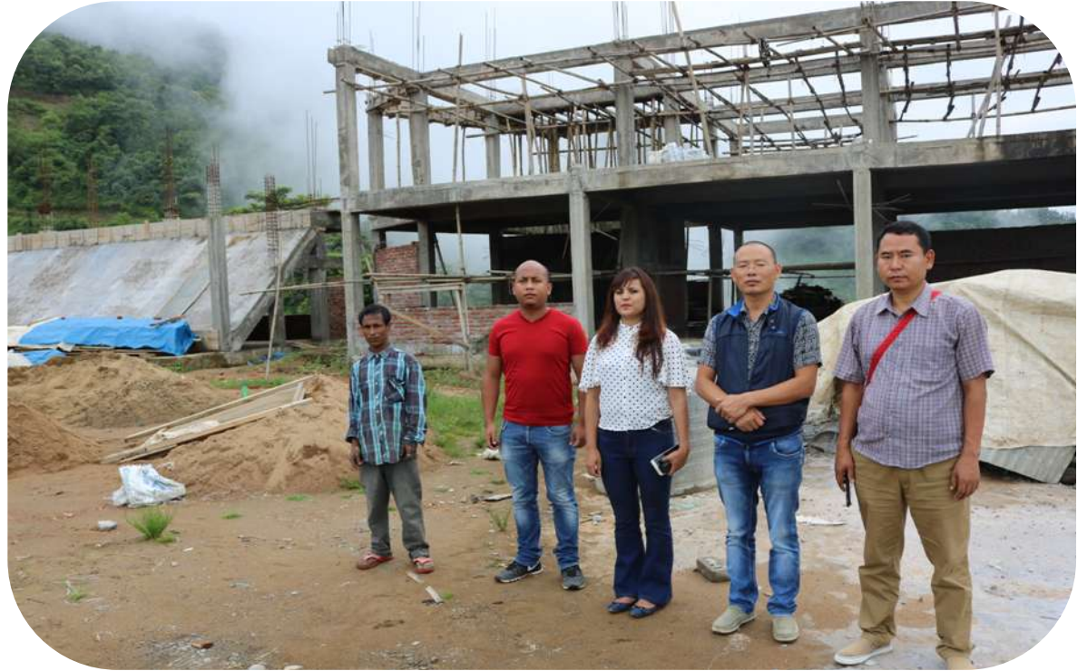
Nec officials with Implementing department at project site.
