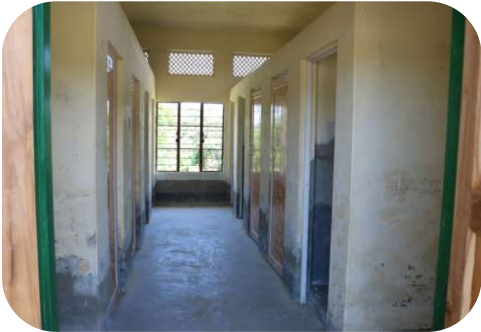
View of Toilet
