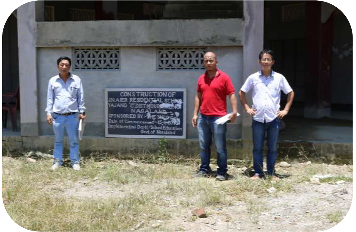
Nec officials with Implementing department at project site.
