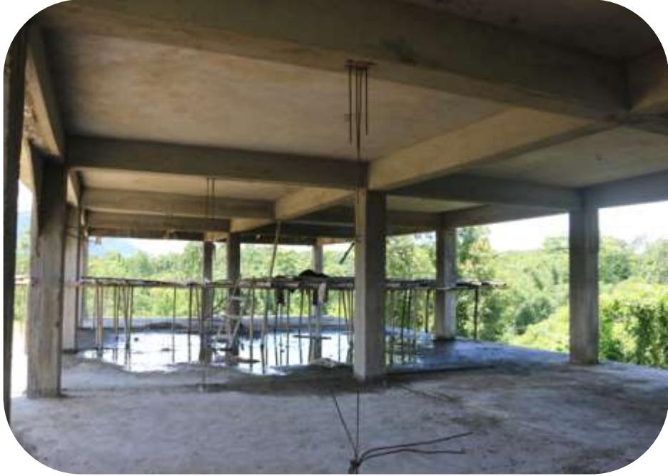
View of Second floor
