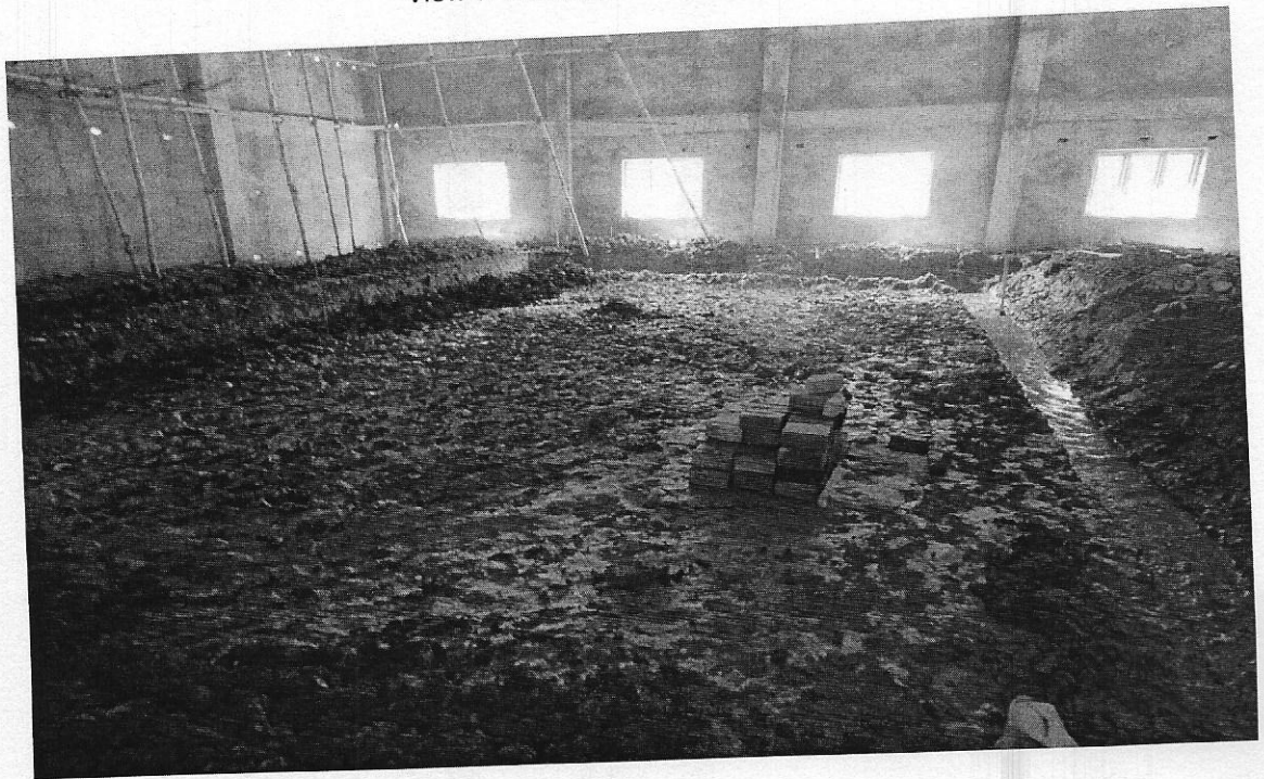
View of preparation for construction of badminton court
