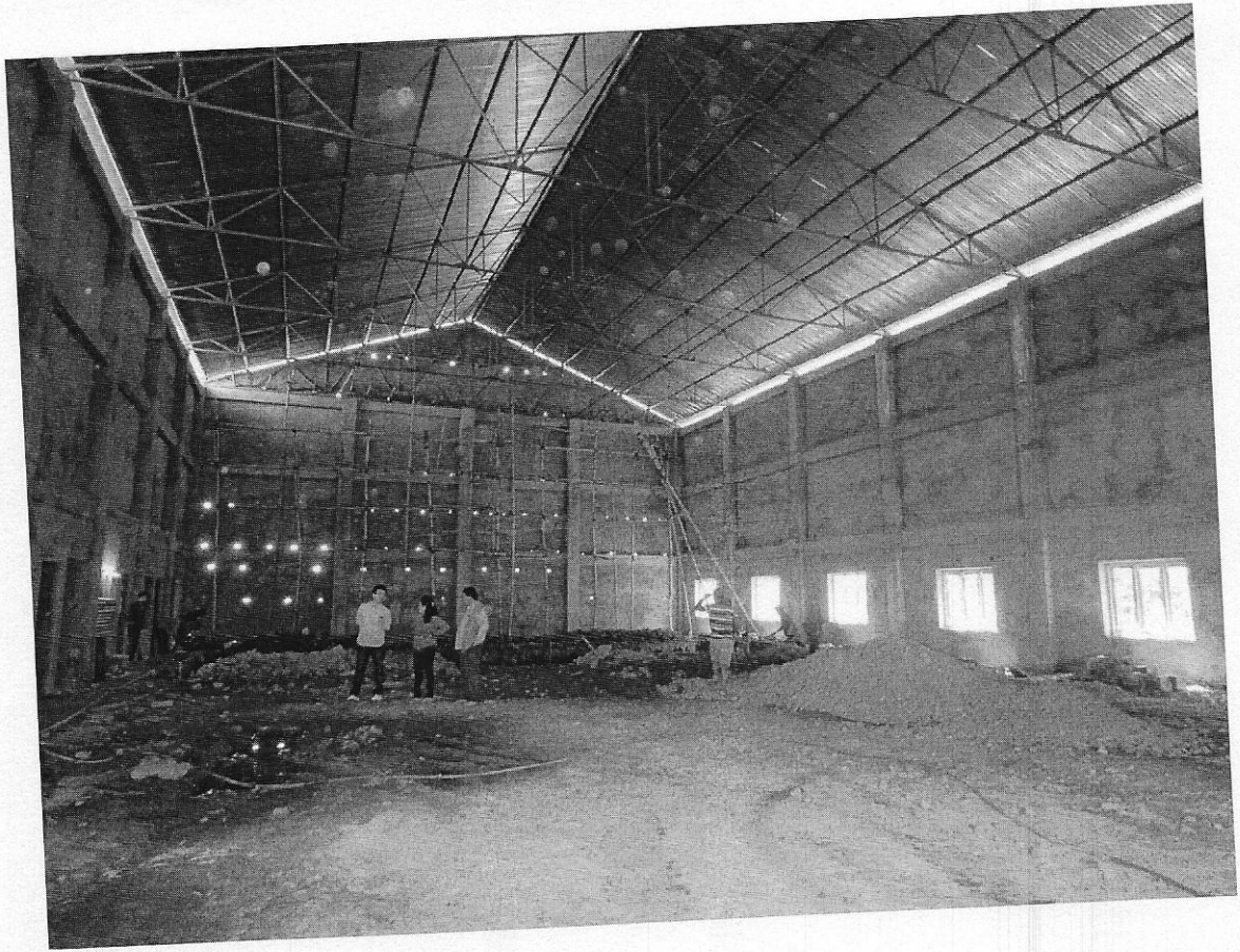
View of inside the indoor stadium
