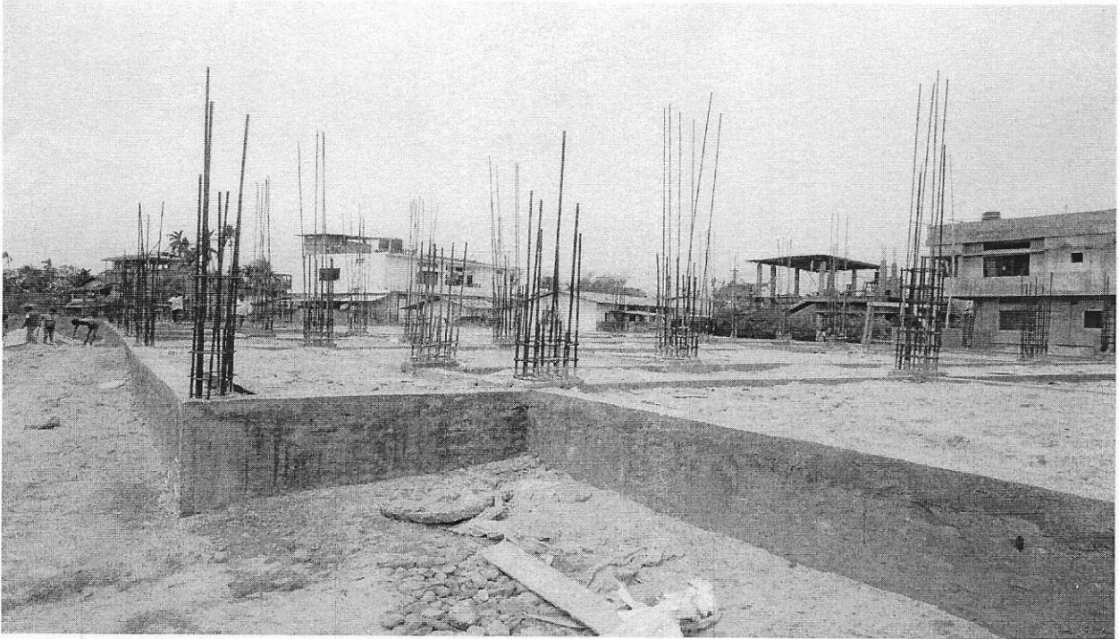
View of the construction work for Community Hall and Auditorium
