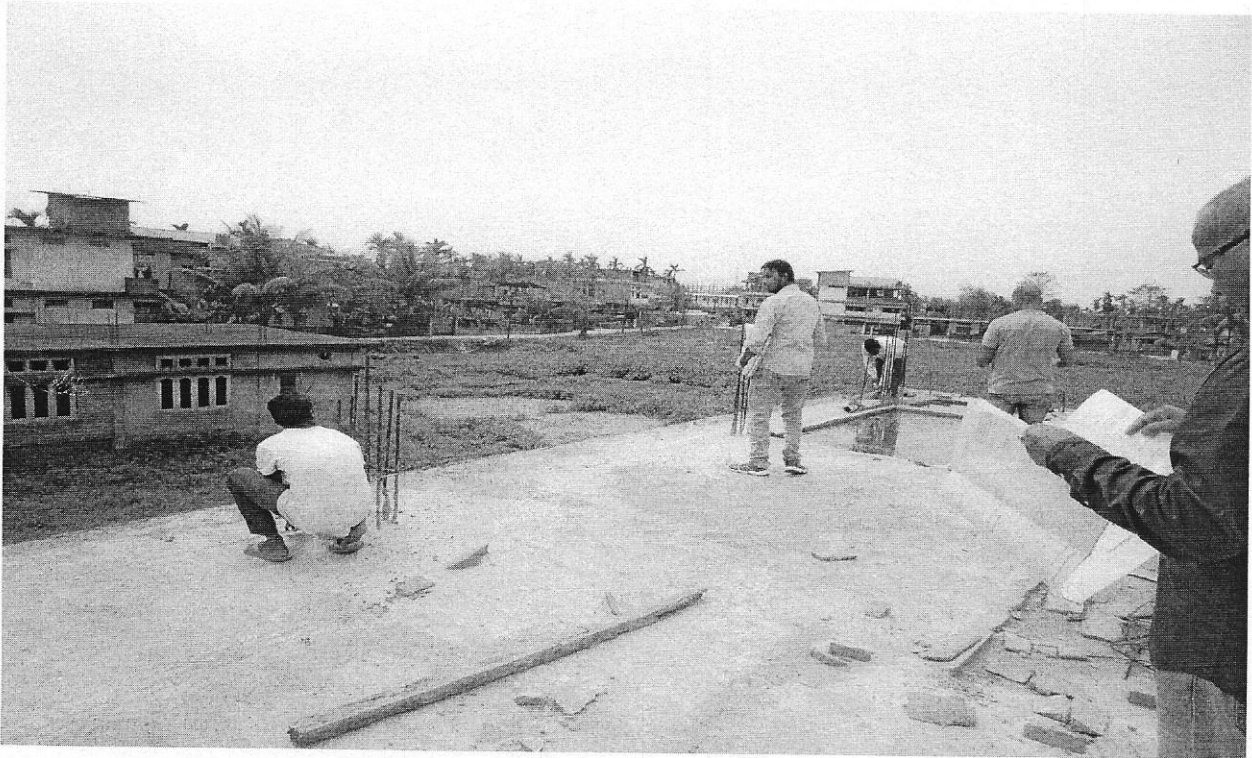
Plinth Measurement taking for the Guest House
