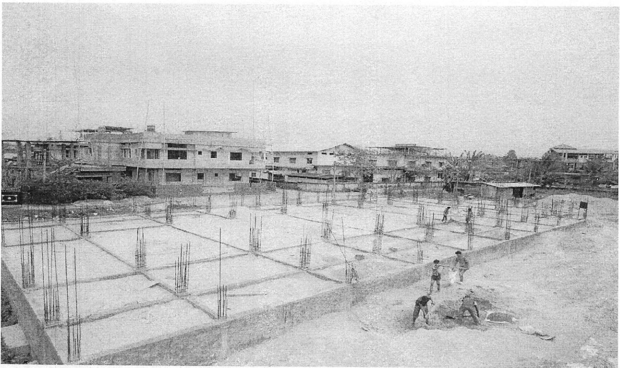
Top View of the construction work for Community Hall and Auditorium
