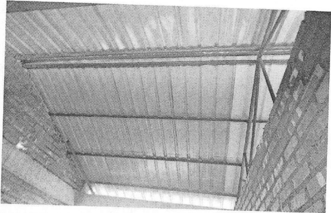
Photo of the truss inside the Girls Hostel
