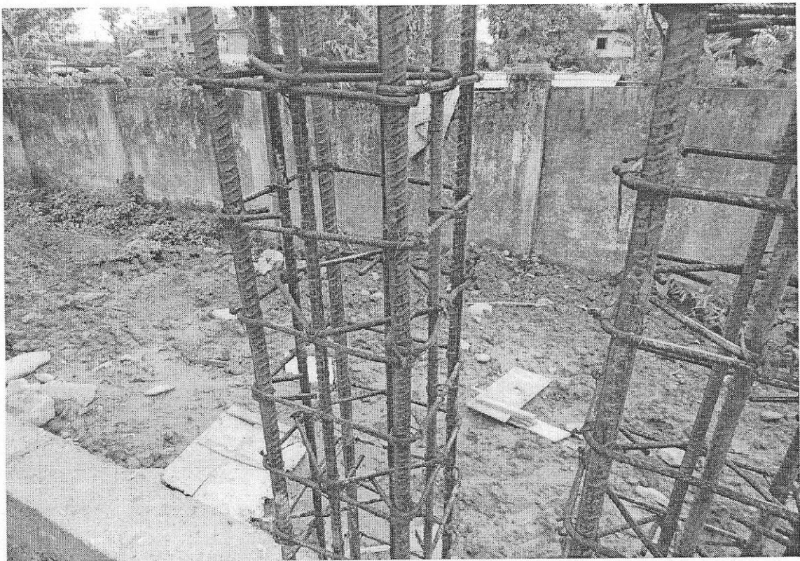
Photo of the reinforcement used in columns
