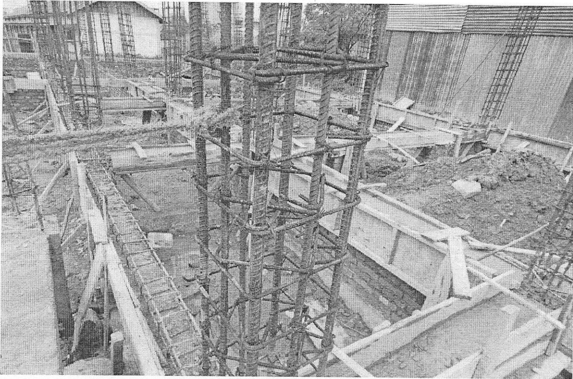
Photo of Plinth beam reinforcements.
