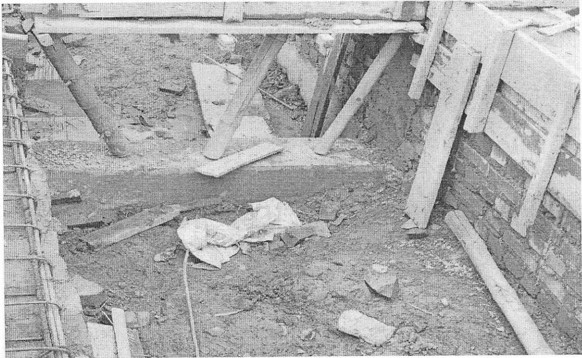
Photo of Grade Beam
