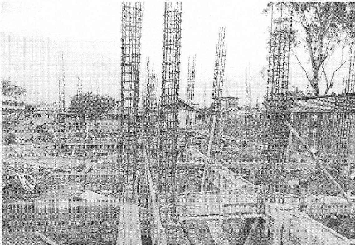
Photo of plinth beam and columns reinforcement.
