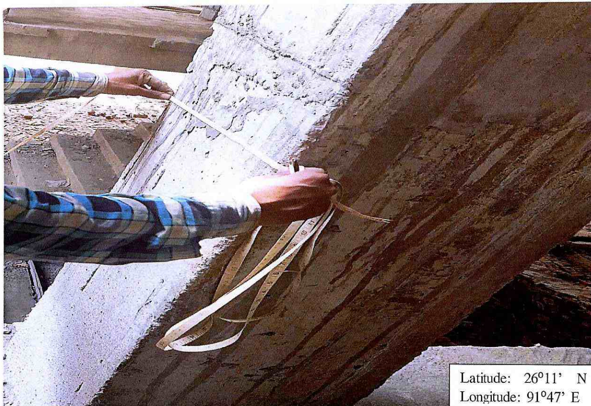
Photo of the inspection team measuring the column of the building for the “Construction of building for the department of Geology in Cotton College”, Guwahati, Assam
