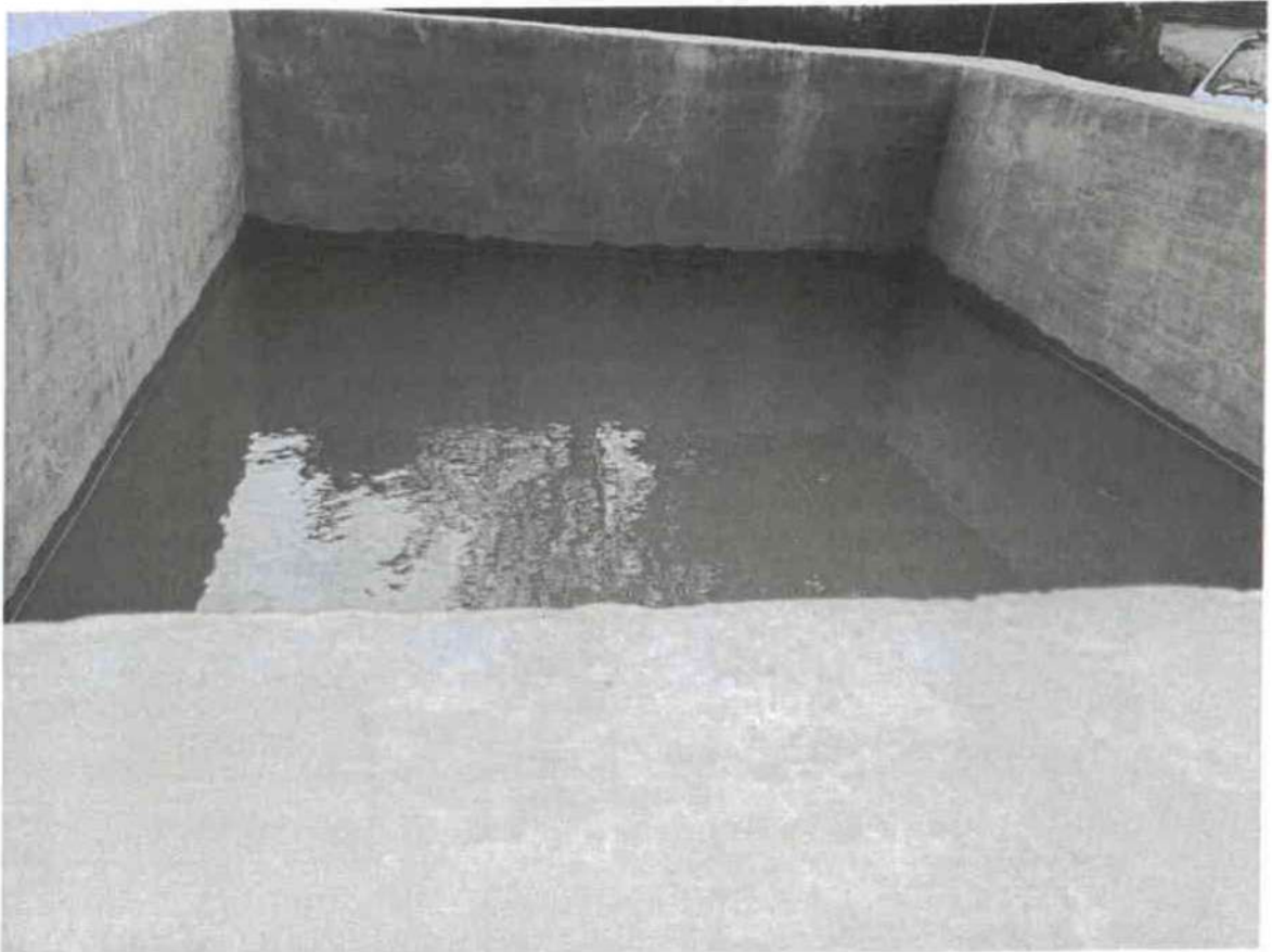
Photo of the borewell and the water tank for the "Installation of borewell at Khusi Tampakvillage" – Location 5
