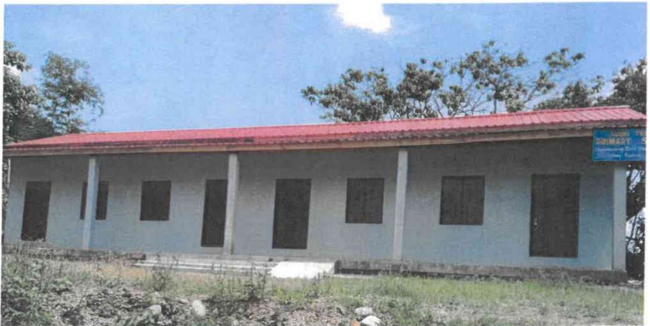
Overall view of the “Construction of Primary School at Sugnu Tribal, Manipur”
