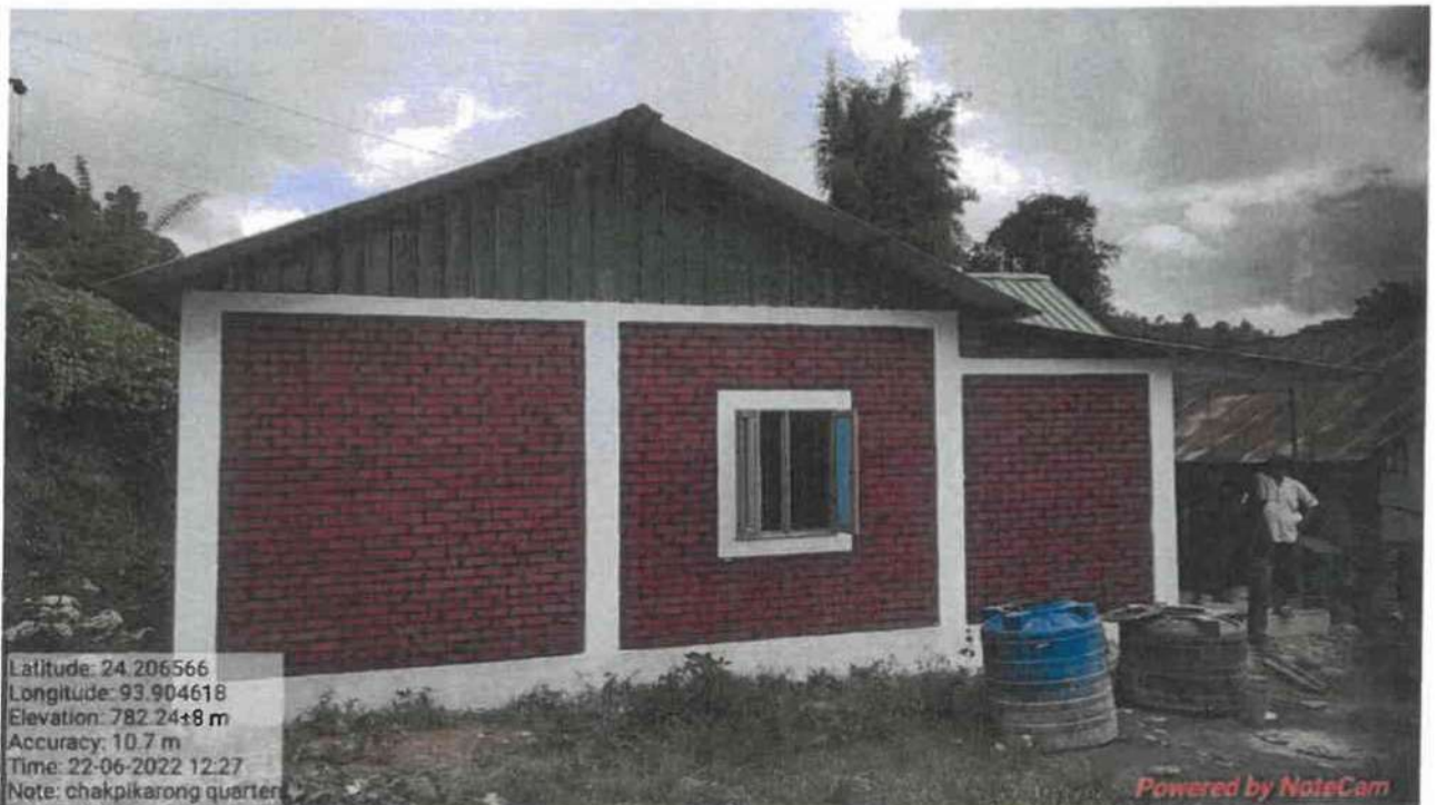
Side view of the “Construction of Teacher’s Transit Quarter at SDO Office Complex, Chakpikarong”
