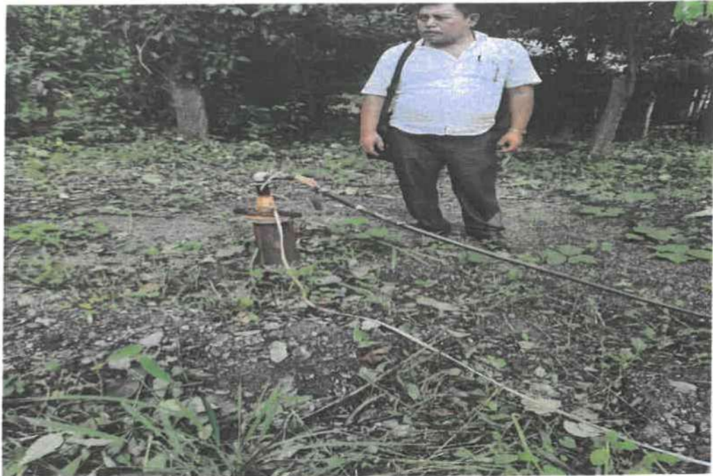
Photo of the “Installation of borewell at Thungcheng village”– Location 7
