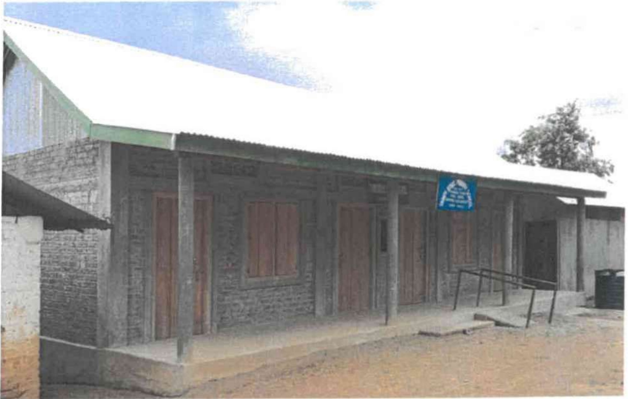
Overall view of "Construction of 2 additional Classrooms at Kovol Primary School, Tami, Manipur"
