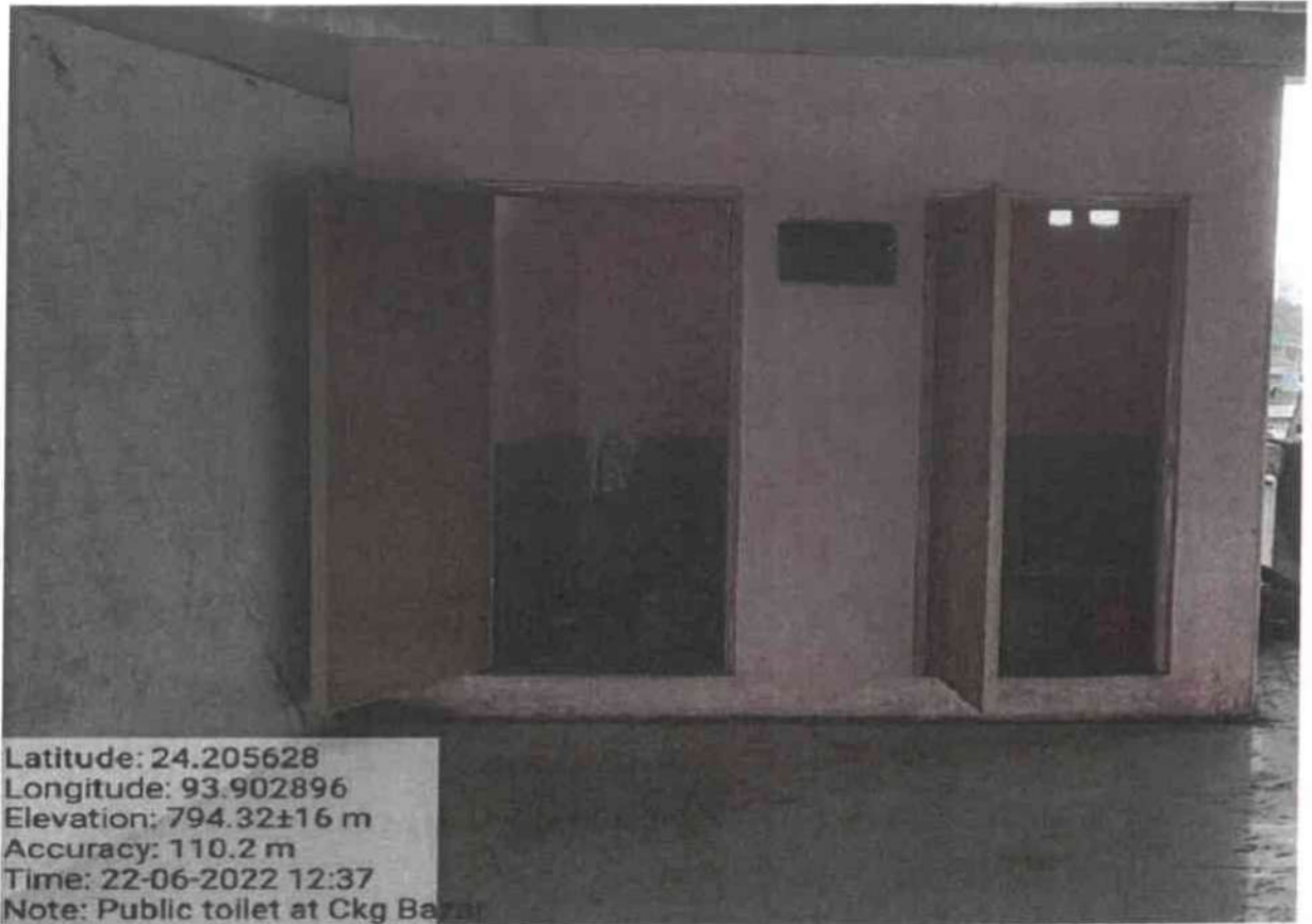
Photograph showing the “Construction of Public Toilet at Chakikarong Bazar, Manipur”
