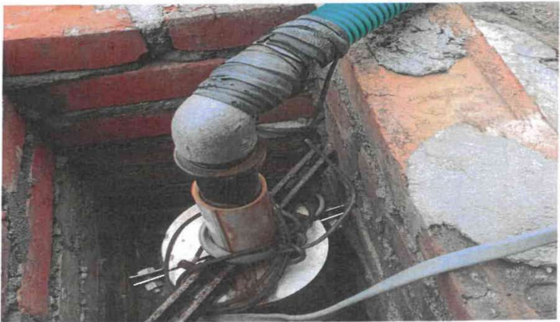
Photo of the "Installation of borewell at Sengul Colony village" – Location 4
