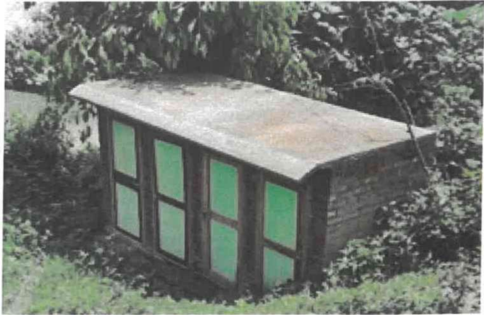
Photo showing the Toilet constructed at "Construction of Primary School at Sugnu Tribal, Manipur"
