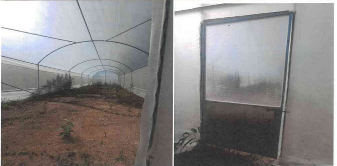
View of the greenhouses installed at Bungmun.
