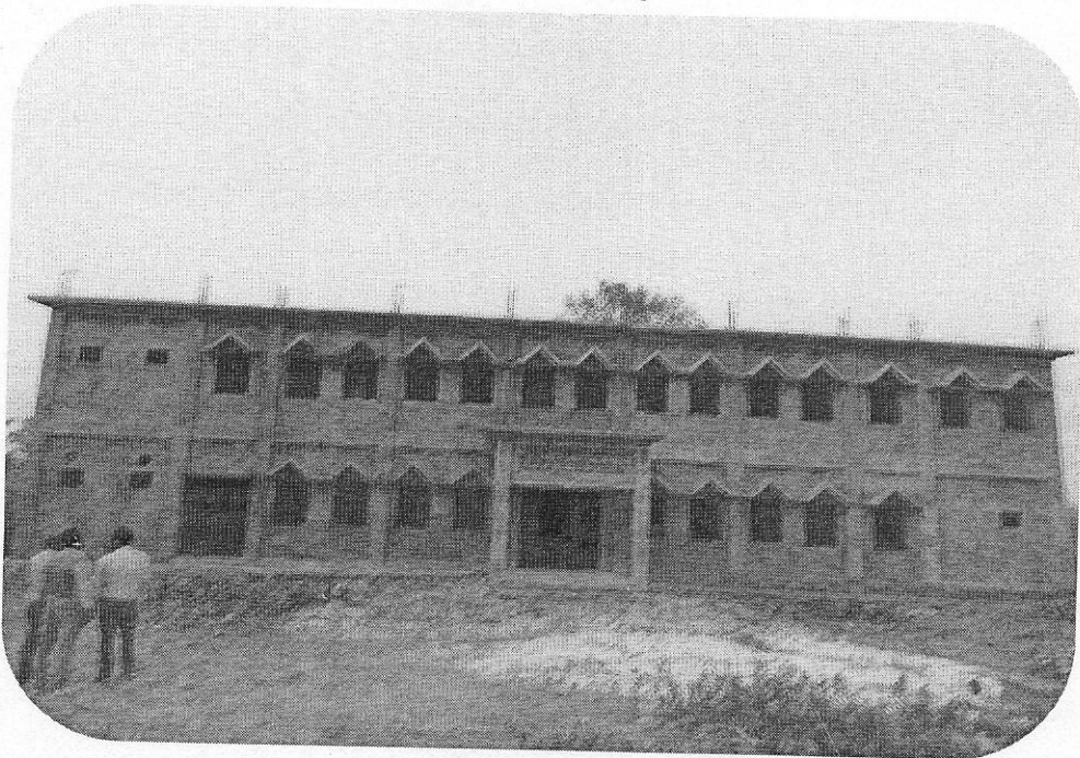
View of Hostel
