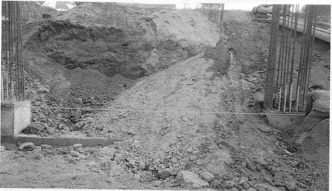
Mesurement taking of the columns spacing of Institute Building Omeo Kumar Das Institute of Social Change and Development
