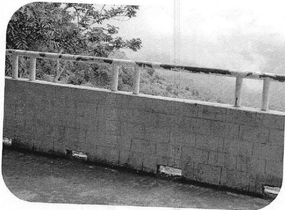
View of security fencing.
