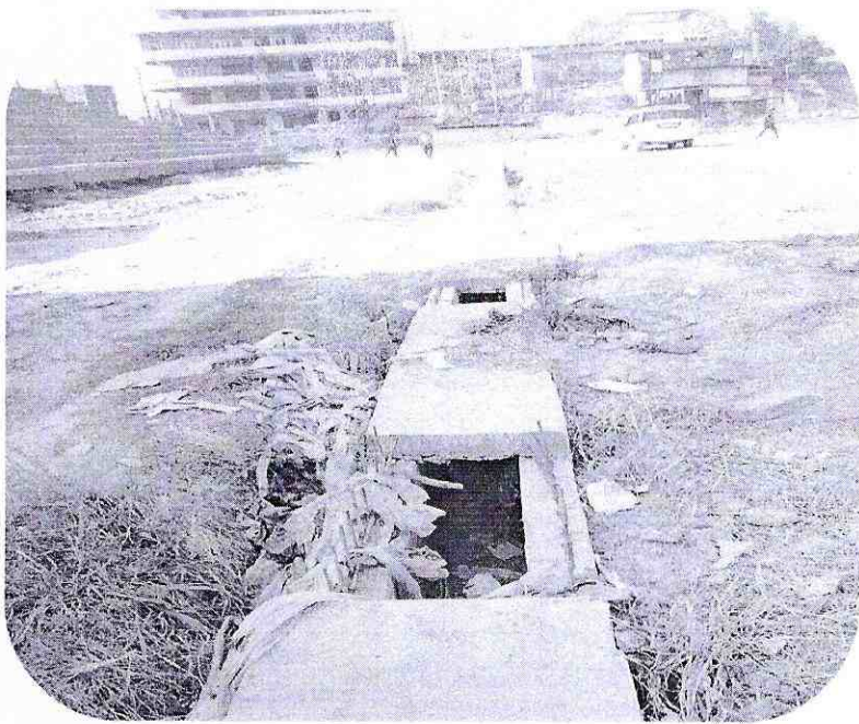
View of drain
