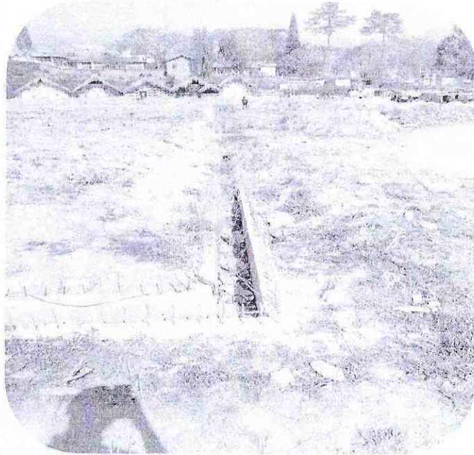
View of drain construction in progress.
