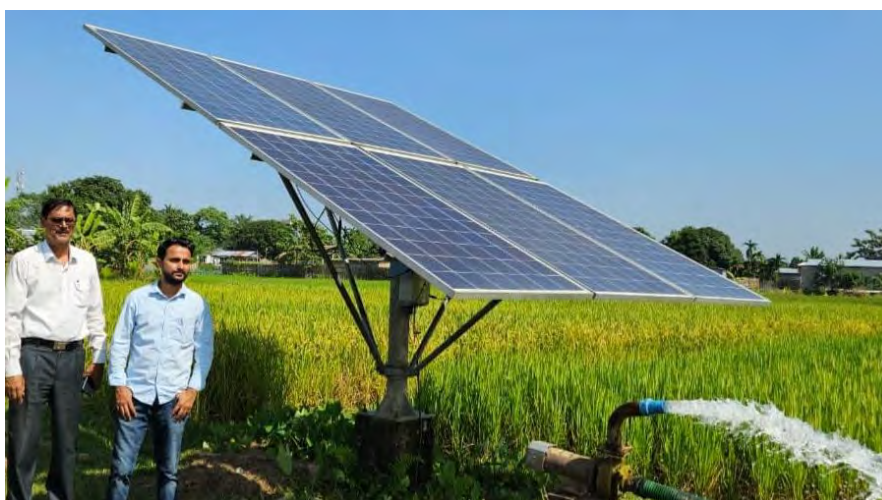
Solar powered pumps have been installed for irrigation purposes at many places in the NE Region
