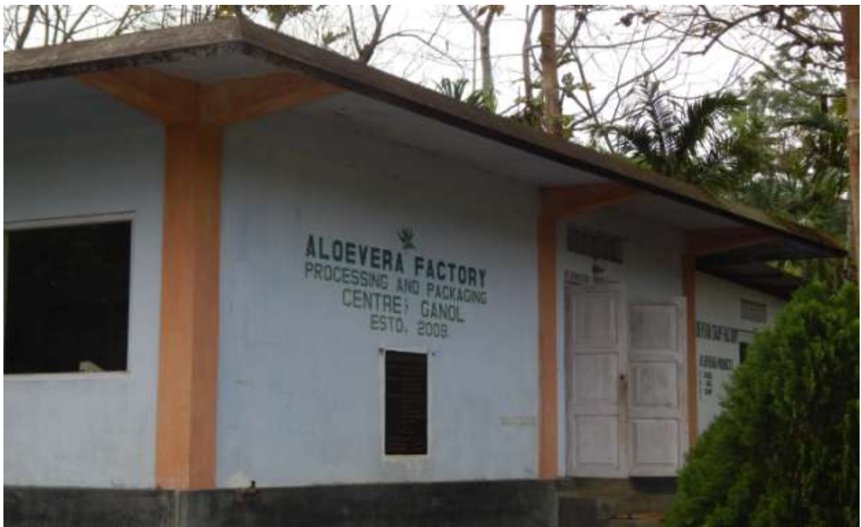
View of Aloe vera Processing and Packing Unit in West Garo Hill
