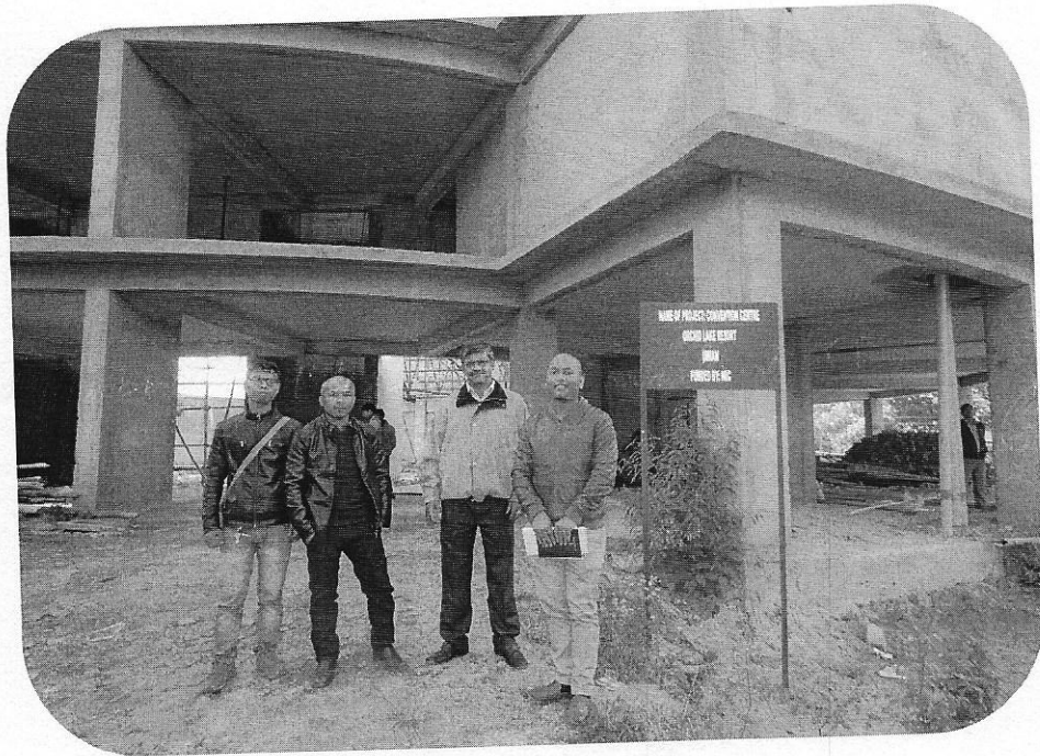
Inspection team with Implementing Agency at project site
