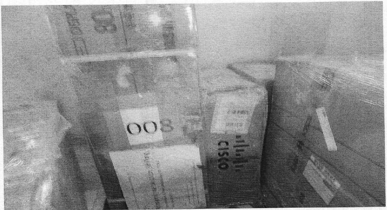
View of material of EPABX System
