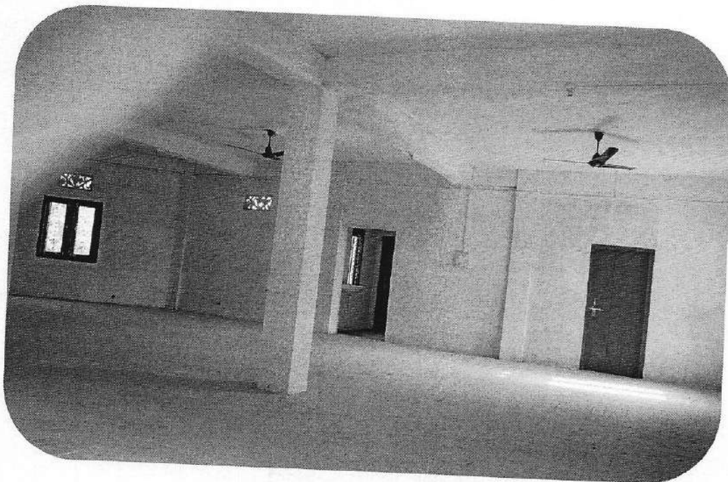
View of inside the cafeteria
