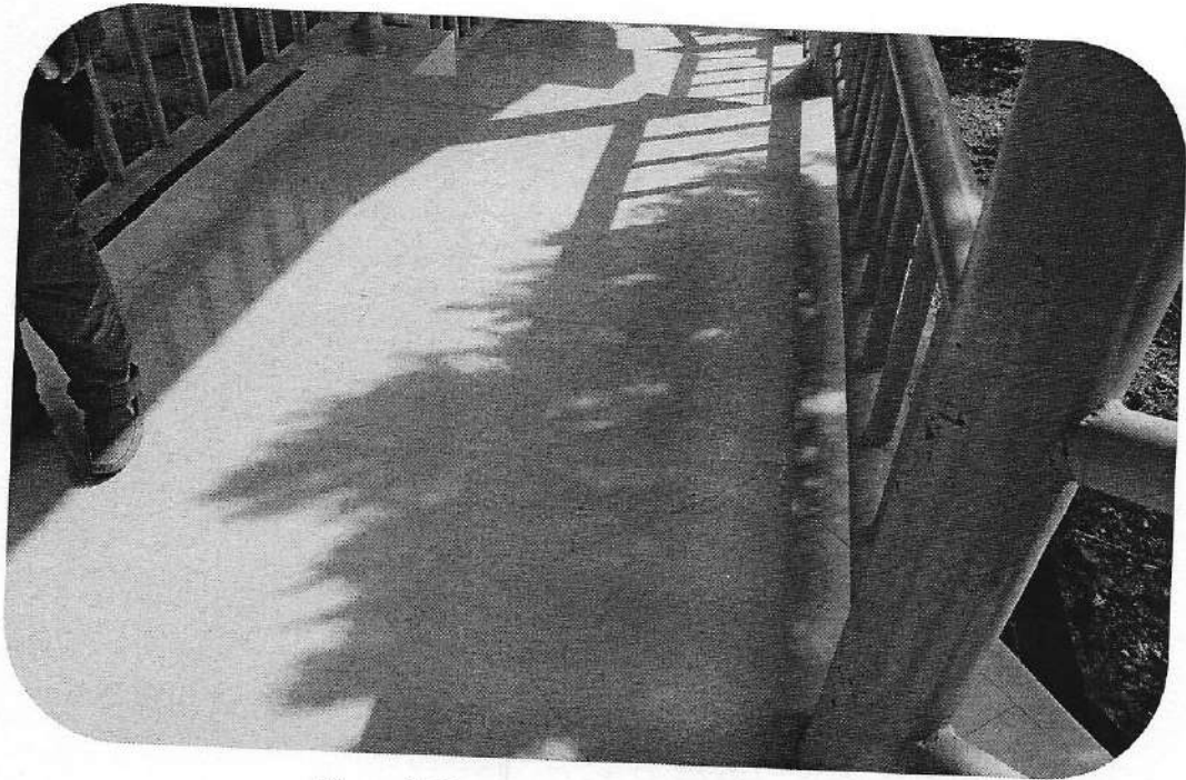
View of Tiles in flooring after renovation
