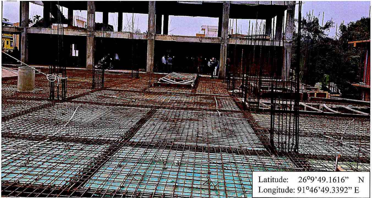
Photo of the ongoing work of the binding of Reinforcement for slab of first floor for the “Construction of Composite Regional Centre(North East) for Disability Study and Action in Assam by Shishu Sarothi”
