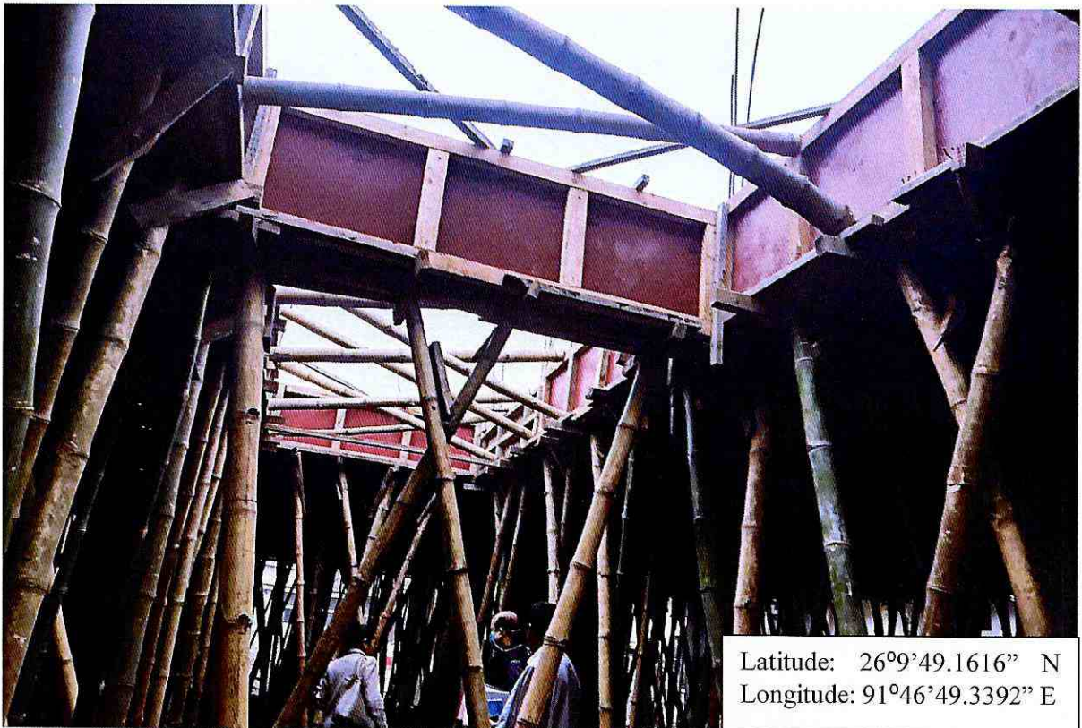
Photo showing the shuttering work in progress for beam in Second floor for the “Construction of Composite Regional Centre(North East) for Disability Study and Action in Assam by Shishu Sarothi”
