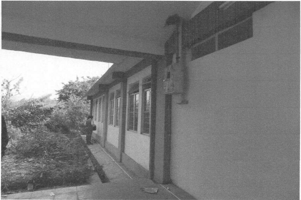
A view of the inspection taking the Plinth Area.
