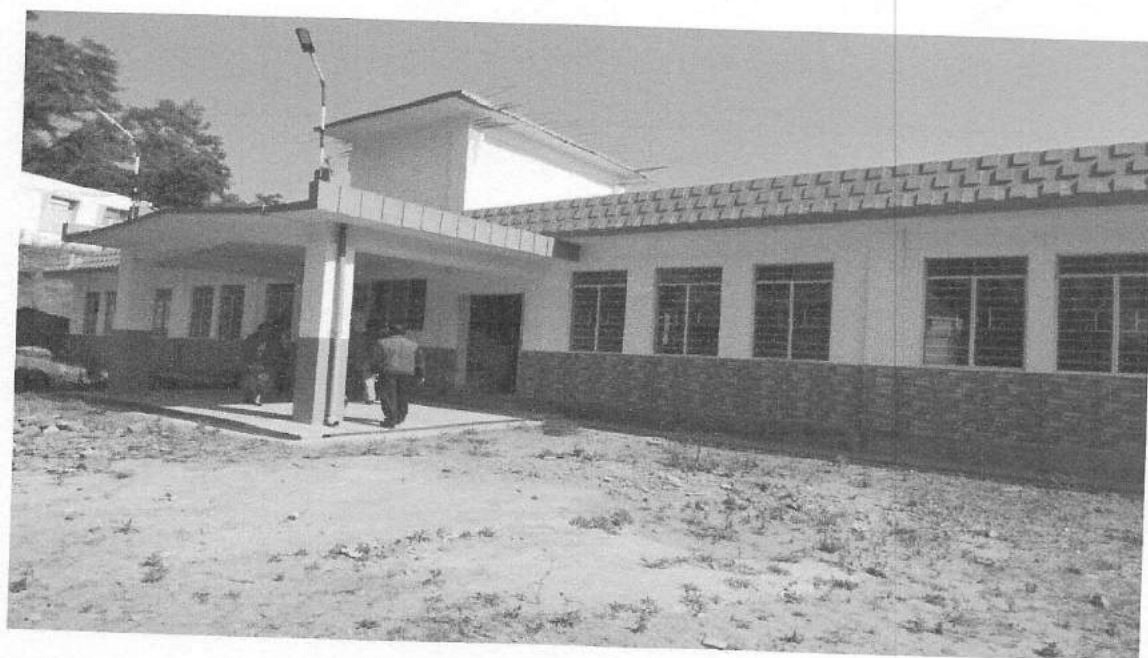
A view of the Inspection Team measuring the Plinth Area.
