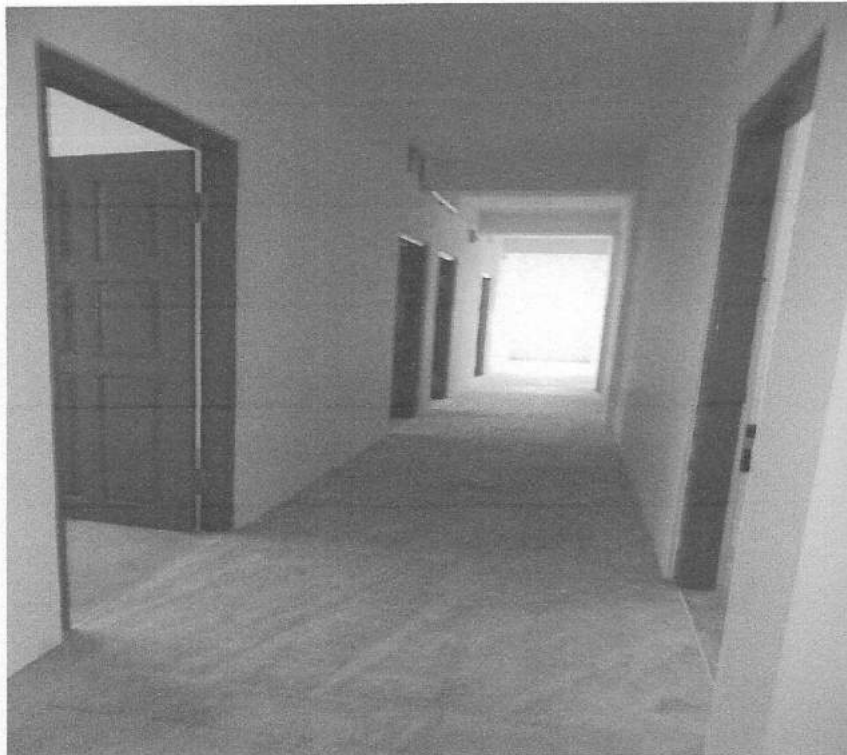
A view of the corridor covered with marbles.
