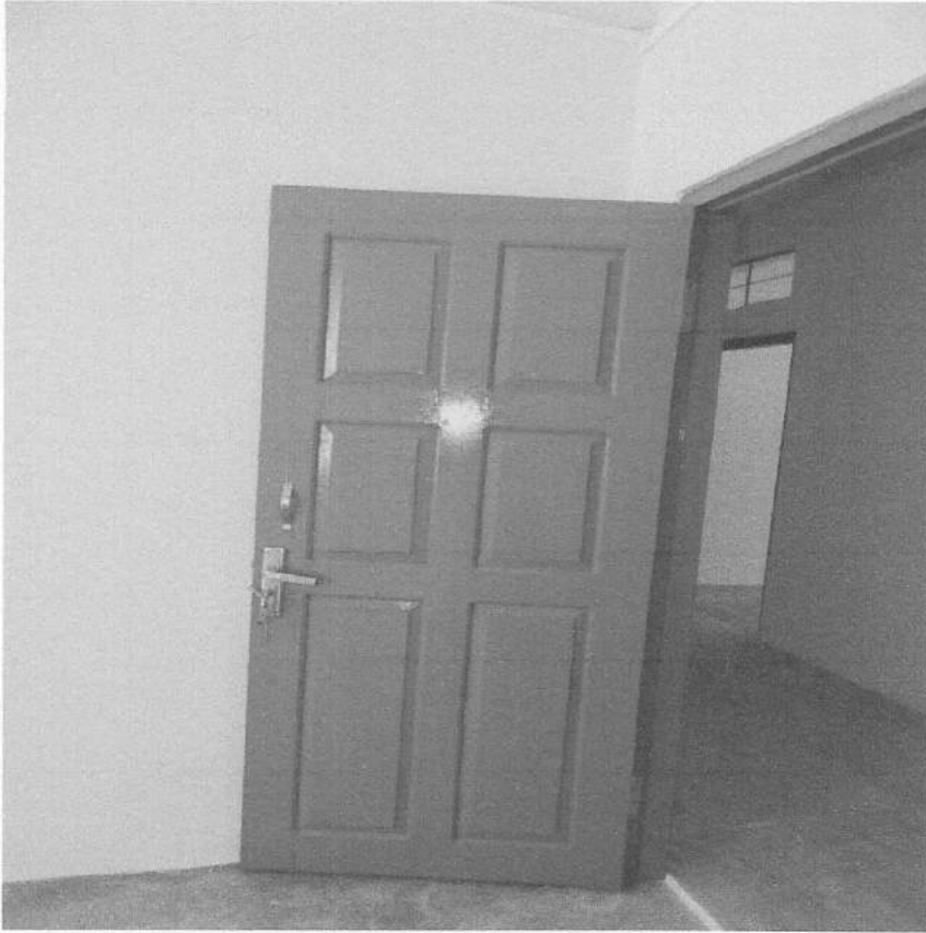
A view of one of the doors.
