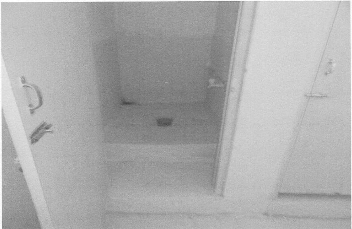
A view of the inside of the common toilet.
