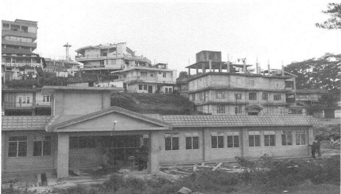
A view of the Inspection Team measuring the Plinth Area of the Laboratory.
