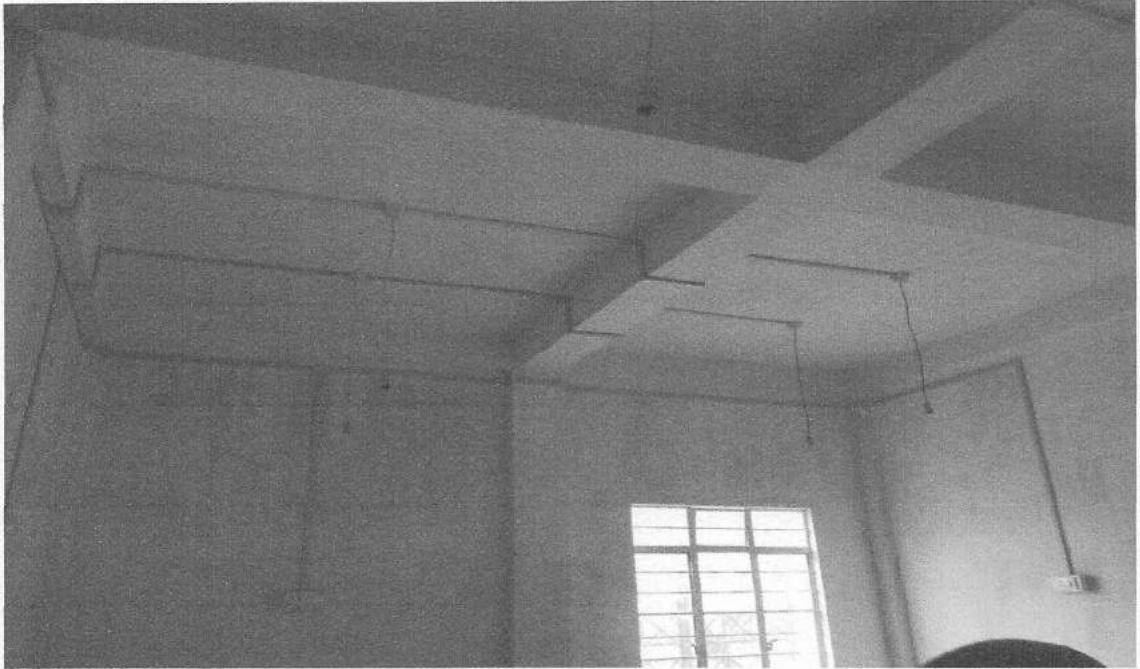
View of electrical work inside the Laboratory.
