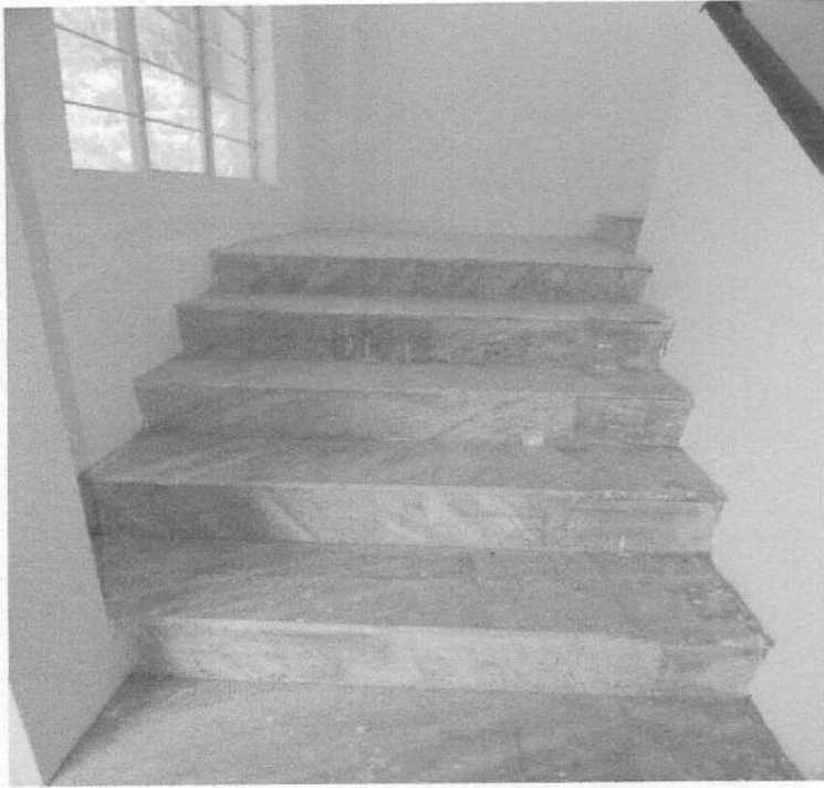
A view of the staircase covered by marbles.
