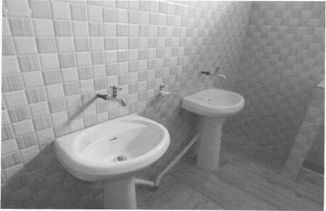
A view of the sink at the common toilet.
