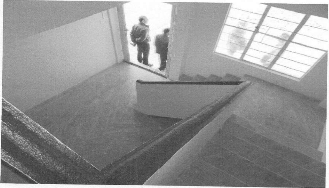
A top view of the staircase and the lobby.
