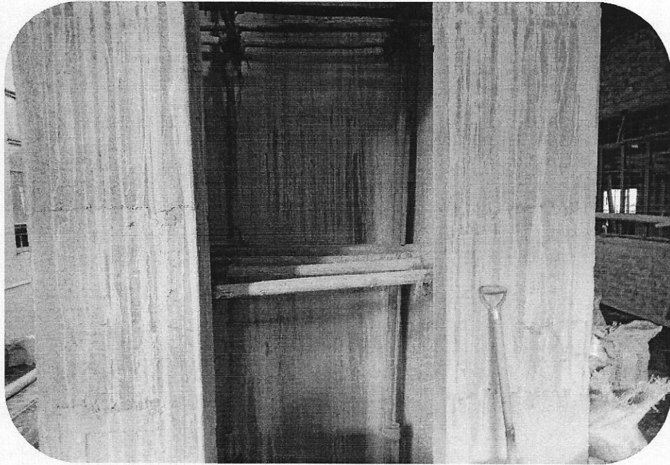
view of Lift well
