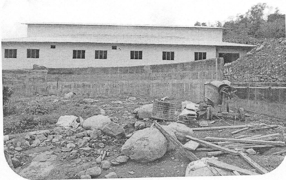
View of retaining wall
