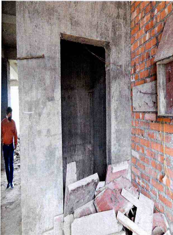
4.View showing the provision of lift system of Multi- Disciplinary Livelihood Incubation centre for Food Processing, Ready Garment making and Handicraft at Hunpun, Ukhrul
