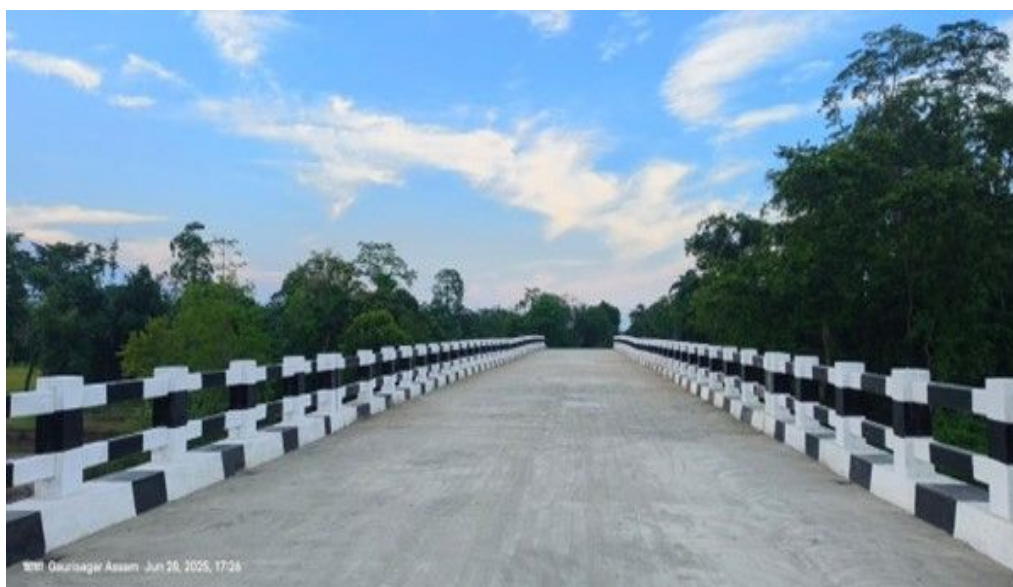
RCC Bridge No. 3/1 over River Dikhow (Road Chiripuria via Ajanpeer Dorgarh) in Assam
