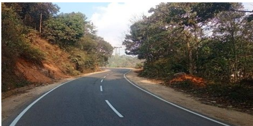
(Completed work: Mawshynrut to Hahim (Athiabari) Road in Meghalaya)
