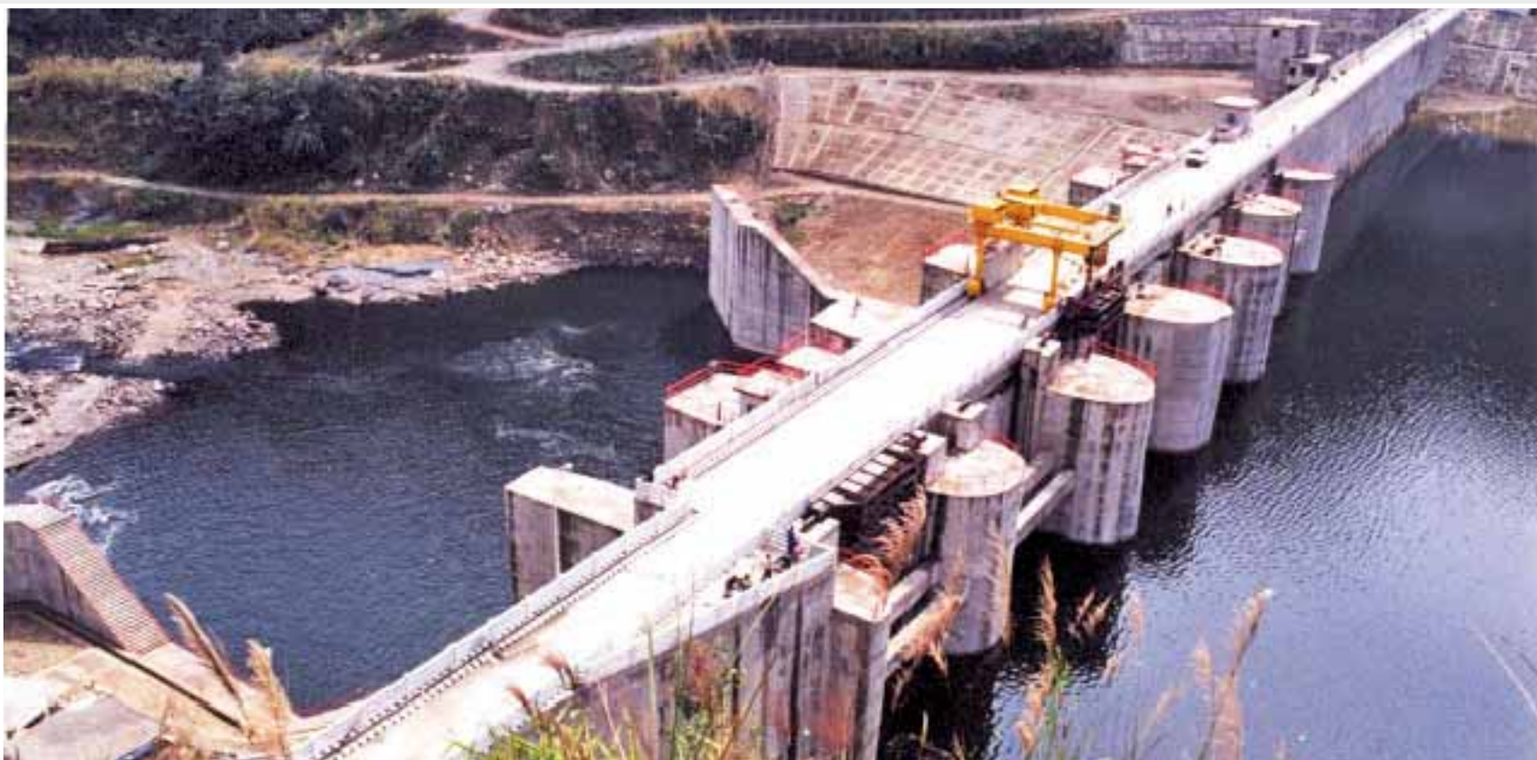
The 405 MW installed capacity Ranganadi Hydro Power Station is a run-of-the-river scheme with a small pondage to harness the hydro power of Ranganadi River, located at Lower Subansiri District, Arunachal Pradesh planned in 1988 and became operational in year 2001.
