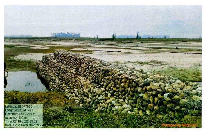
The project was sanctioned during the year 2021-22 at an estimated cost of Rs. 346.53 lakh. NEC has released its entire share in two instalments. The project involves construction Gabion walls/ structures to protect the affected villages of Sigar, Motum, Borguli and Seram under Mebo Block from continuous erosion from the flush flood waters of the river Siang. The physical progress of work is 100%.
