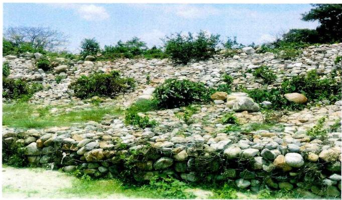
The project was sanctioned during the year 2020-21 at an estimated cost of Rs. 495.73 lakh. NEC has released an amount of Rs. 437.27 lakh. In order to prevent flood and erosion problems in the Darranga area at different reaches, anti-erosion measures in the form of boulder filled apron in cage and bank pitching have been provided. On completion, the project will benefit an area of 2500 Ha and a population of about 50,000 nos in 8 villages. The physical progress of work is 100%.
